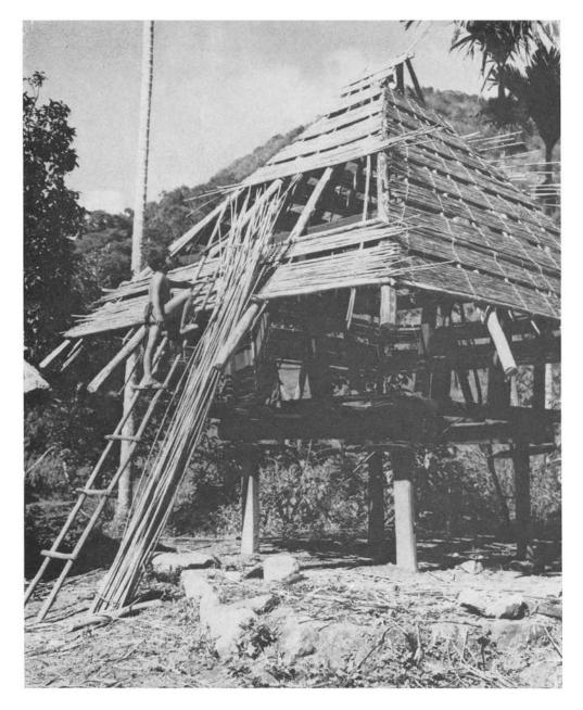
Fig. 3. Roof frame construction showing the use of *Miscanthus* cane grass (*bilāu*, [32; 42]) stems; Bayninan, 1962.
