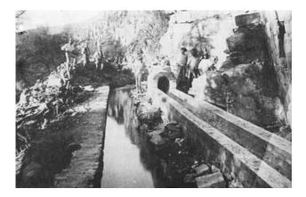
**Figure 10.** Construction of the Mackie's Pit culvert, 1884. Photo: Graaff-Reinet Museum.
