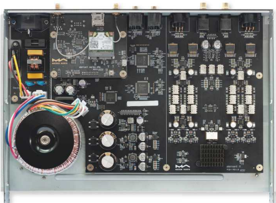
RIGHT: A substantial linear PSU [lower left] has separate regulation for the quad-core ARM CPU [top left], XMOS and Xilinx processors (USB/MQA) [centre], ESS Sabre 9038Pro DAC [lower right] and headphone amp [top right]
