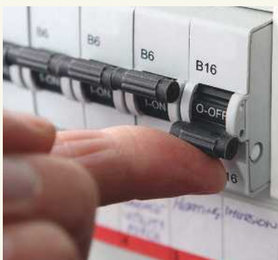
ABOVE: A Miniature Circuit Breaker on a UK domestic electrical consumer unit
