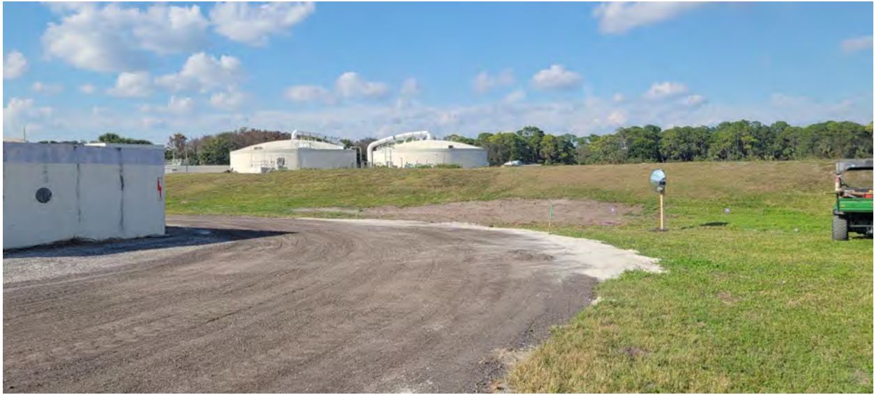
Site Access Driveway Improvements Adjacent to Construction Barn – Looking North
