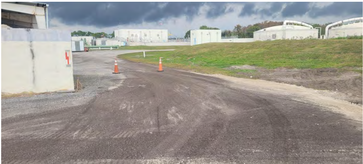
Site Access Driveway Improvements Adjacent to Construction Barn – Looking West
