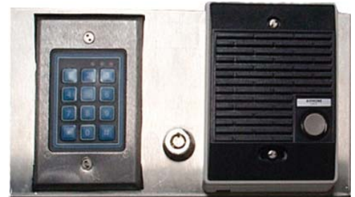
Install a keypad & intercom.
