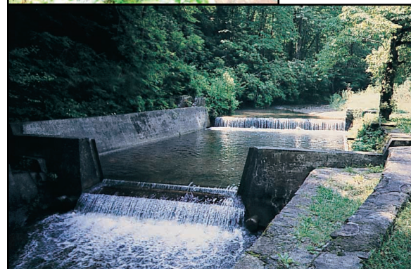
Lotic Inter-site Nitrogen Experiment (LINX): 15 NH 4 additions are made to streams to determine NH 4 uptake length and uptake rate, nitrogen turnover rates, and food web transfer of nitrogen. Pictured here are weirs on Mack Creek at the Andrews LTER site (left) and on Ball Creek at the Coweeta LTER site (below).
