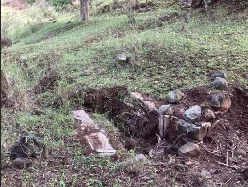
Figure 76. Site 7346 Feature 156-B outflow sluice.
