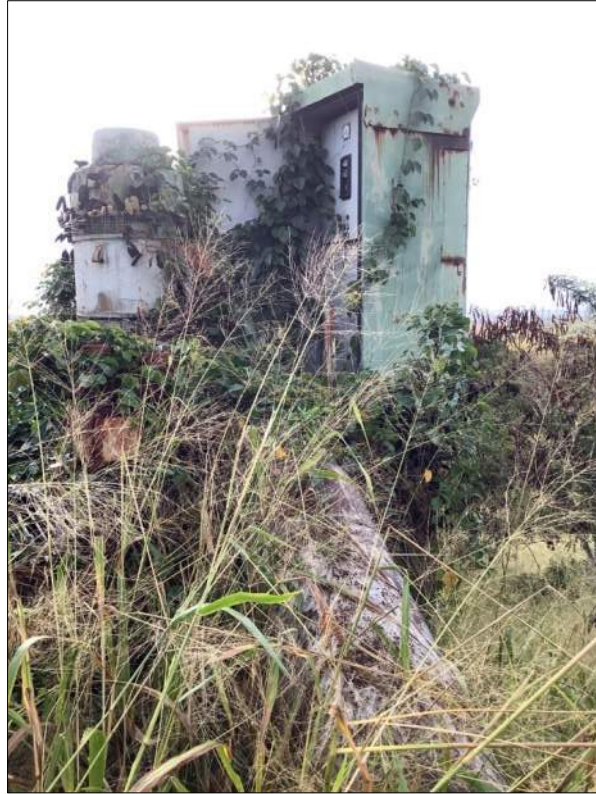
Figure 83. Pump house and siphon.
