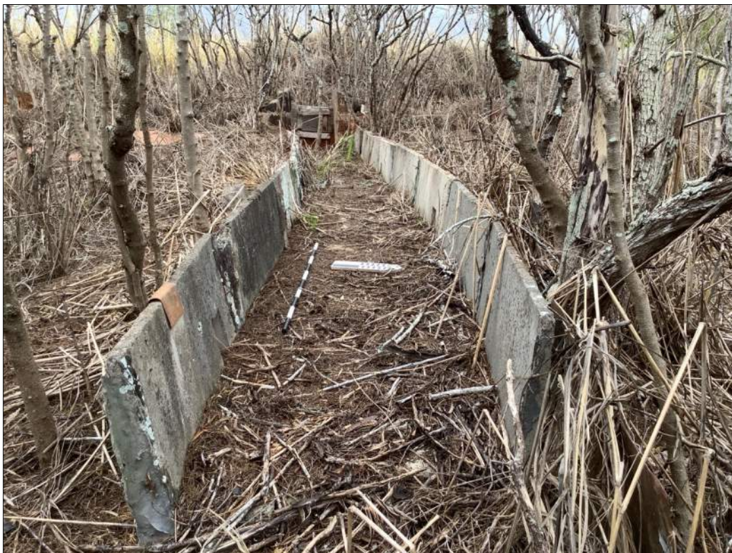
Figure 51. Site 7346 Feature 155-D, western portion of intact flume alignment, view to the west.
