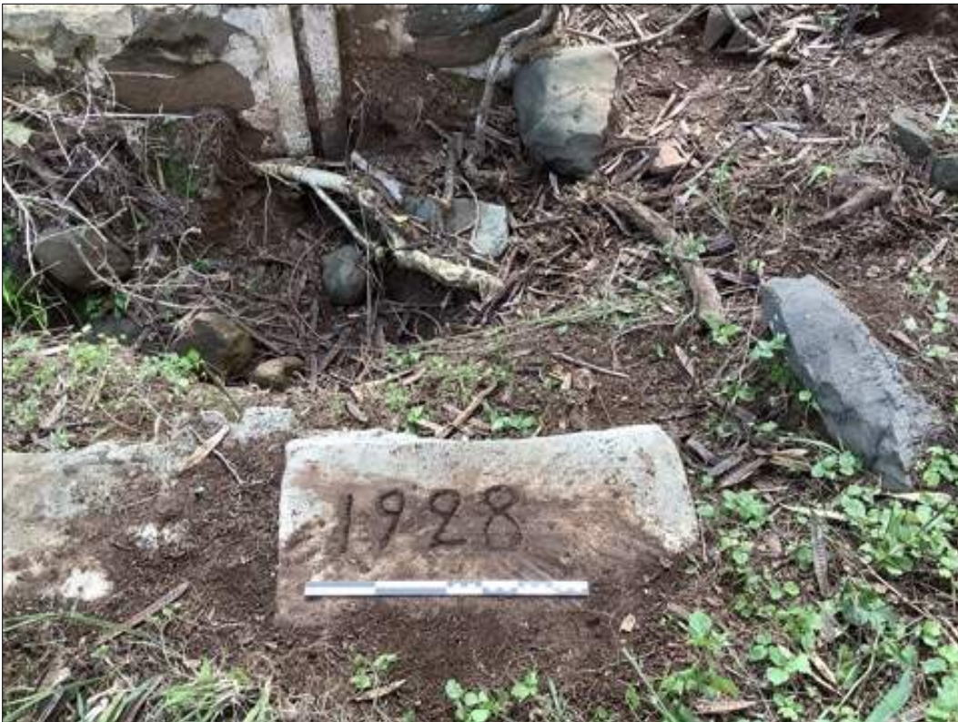
Figure 77. Date (1928) etched in to concrete on Site 7346 Feature 156-B outflow sluice.
