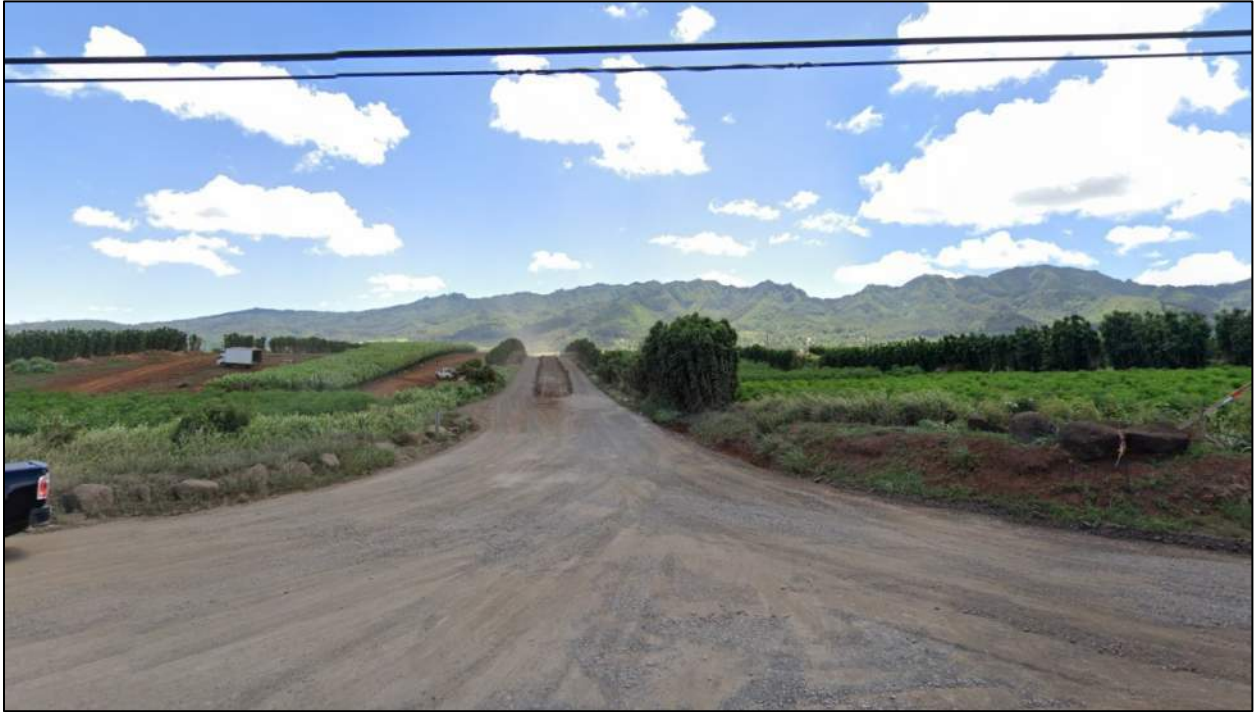
9. Site Access #3, Looking West (June 2019)
