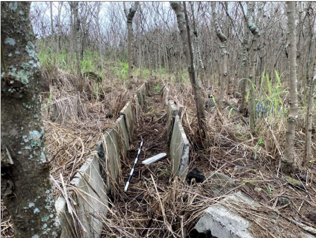
Figure 69. Site 7346 Feature 155-M, southernmost intact section, view to the northwest.
