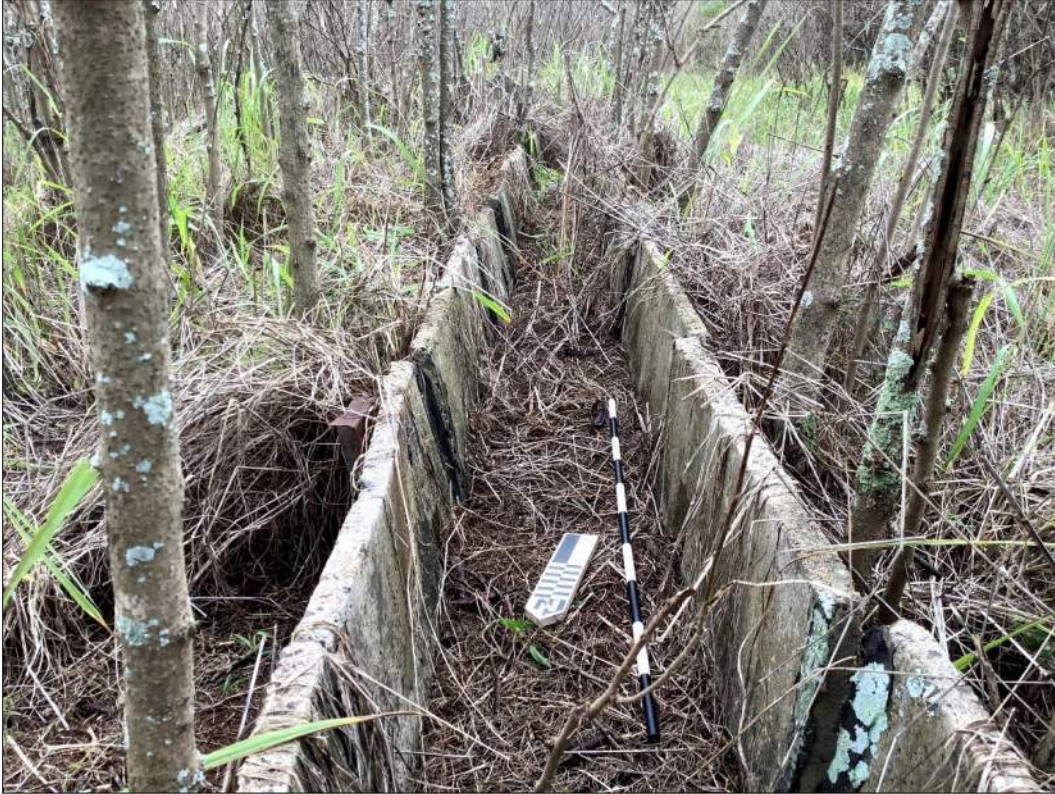
Figure 66. Site 7346 Feature 155-M, northernmost intact section, view to the south.
