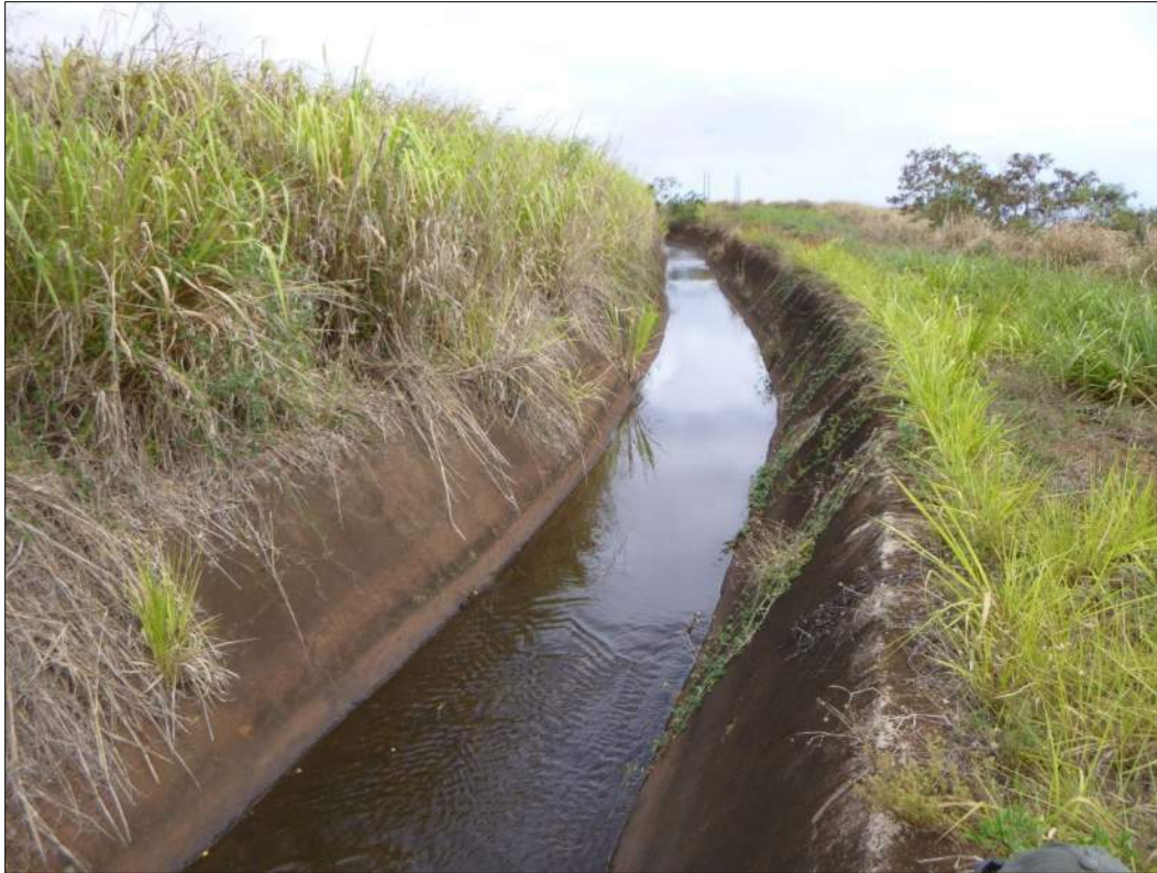
Figure 41. 1916 concreted section of the Waiāhole Ditch.
