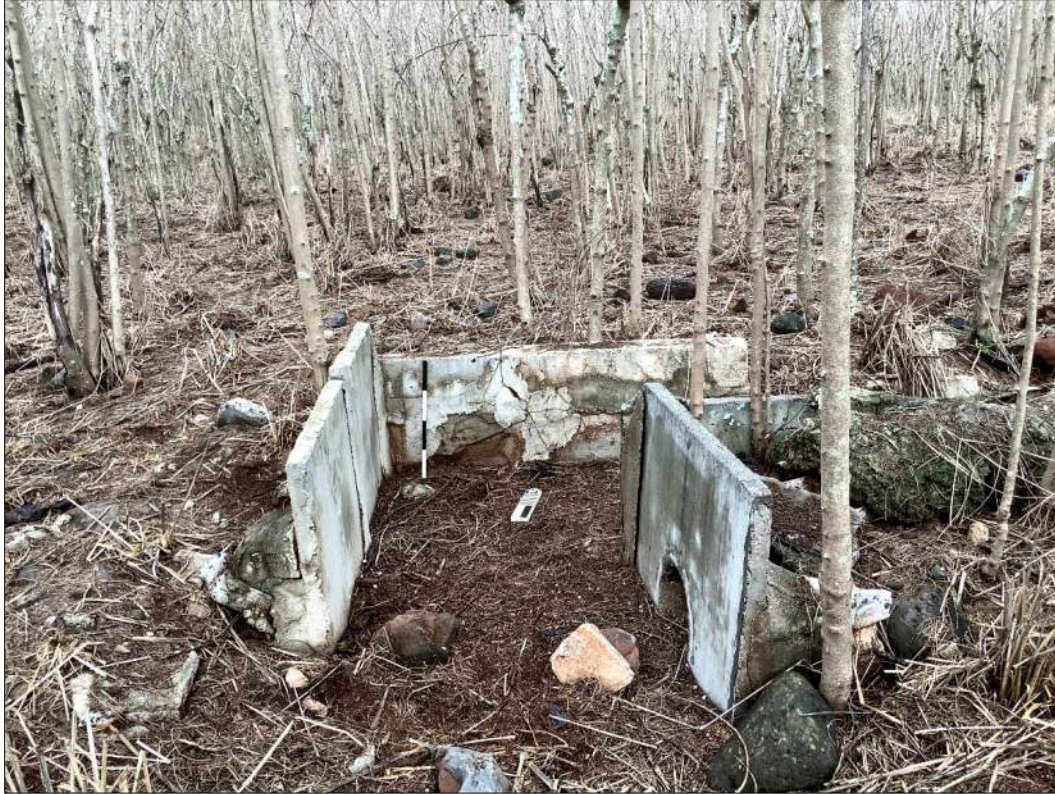
Figure 65. Site 7346 Feature 155-L, 90-degree turn at southwestern end of the flume alignment, view to the north.
