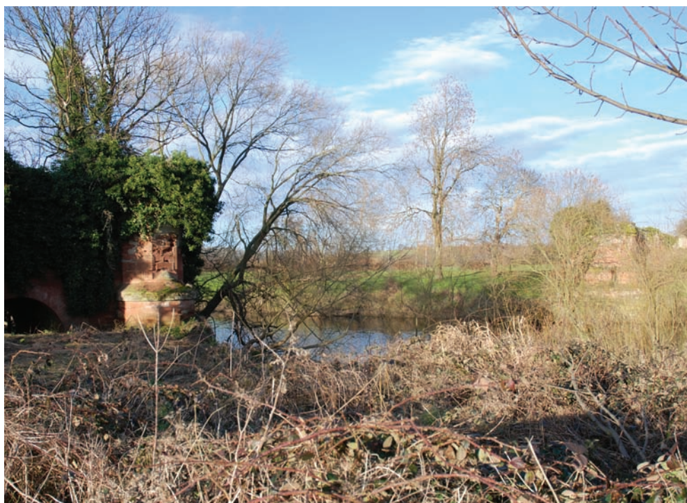
Figure 27. The western bridge abutment viewed from the south. (© C J Dunn)
