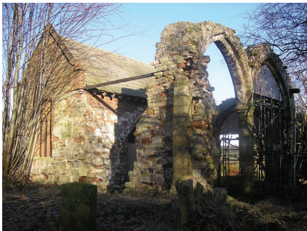
Figure 6. The ruined nave of All Saints' Church showing early stonework in the form of the massive alternative quoins at the north-west corner, bonded to the Conyers Chapel in the 14th century. The south wall is pierced by a 12th-century arcade to the former south aisle
