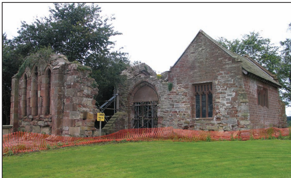
Figure 8. All Saints' Church viewed from the north east in 2007, showing the isolated west chancel wall, the preserved chancel arch and the restored Conyers Chapel
