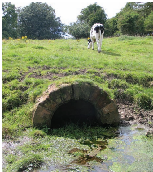
Figure 25. The spring-head vault (feature 27) located between the courtyard and the river
