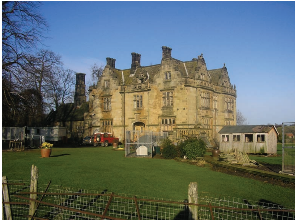
Figure 14. Sockburn Hall viewed from the south west
