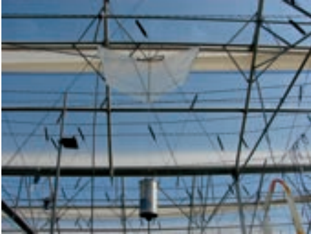
Photo 1. View of a sulphur sublimator
