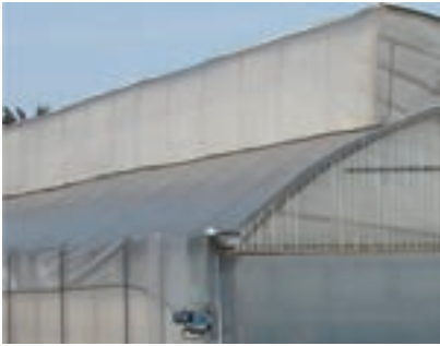
Photo 11. Greenhouse with natural ventilation
