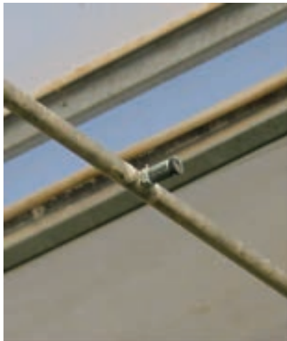
Photo 13. High pressure nebulisation nozzle
