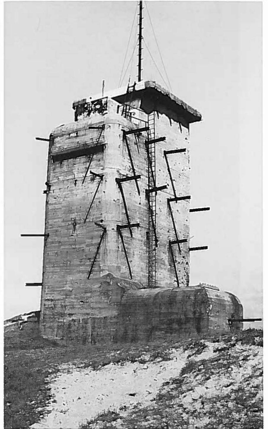
Firing direction tower in Brittany: The steel beams sticking out of this bunker are there to provoke premature explosion of projectiles before they hit the fortification.
