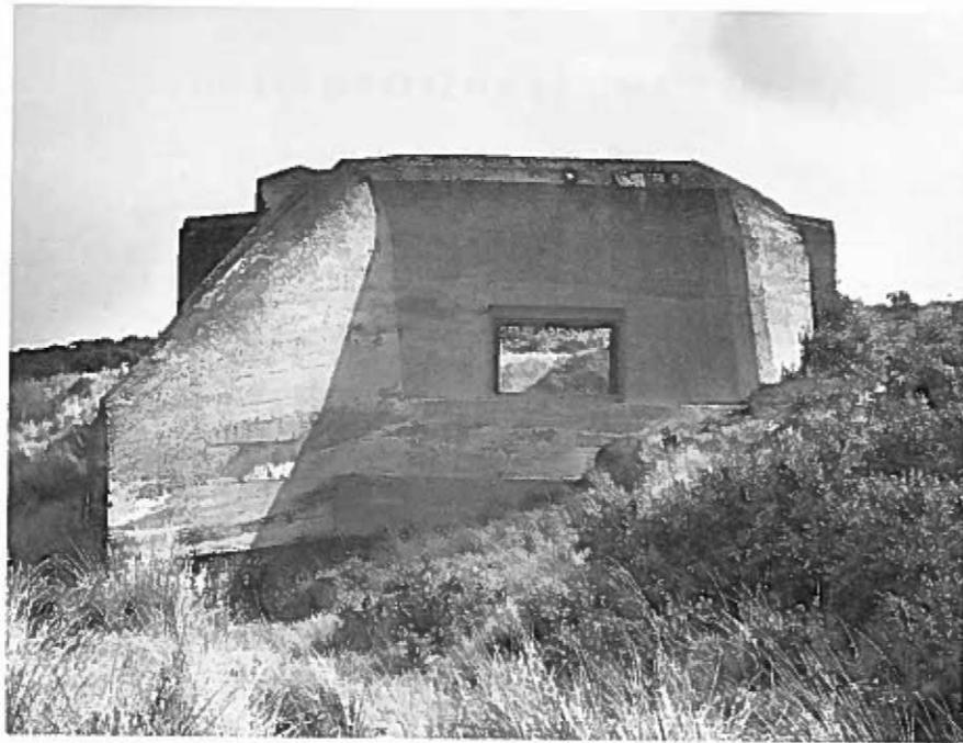
Two types of embrasures for light artillery guns: The graded embrasure avoids the funneling effect. One also notices the concrete material designed to disguise the fortification.
