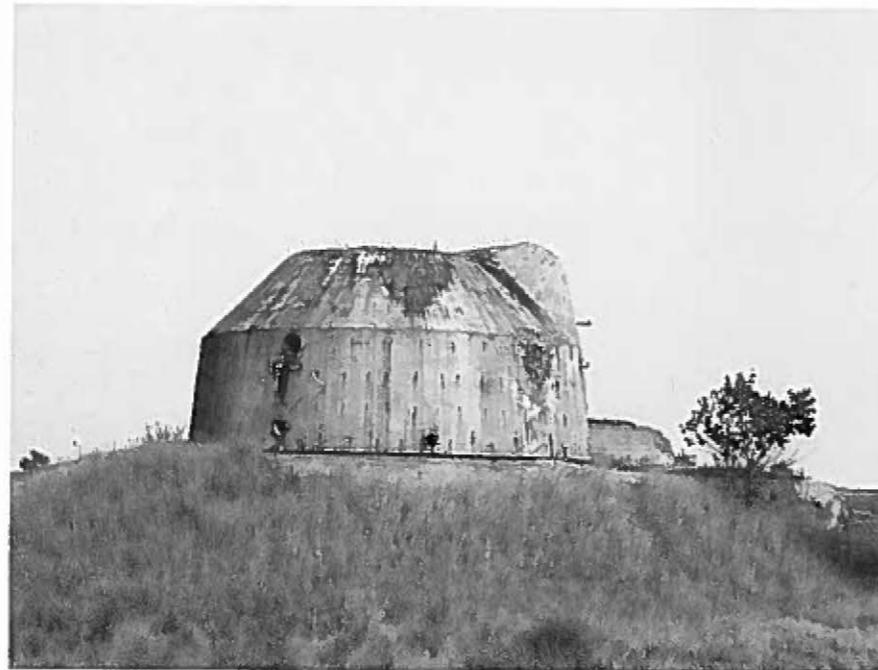
Experimental mobile bunker: The upper mass pivots on its base and shows alternately its open face during firing and its blind side for protection after firing.
