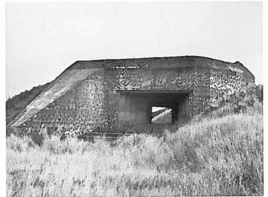
The smooth embrasure signifies that the fortification will get armor plating. The inclined mass, existing in each bunker, serves to screen it and to mark the cannon's blind spot.
