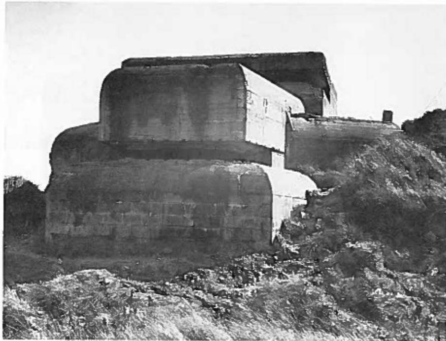
Two types of facades: The upper slab protects the telemeter, which controls the firing in the battery; the lower slab protects the command.
