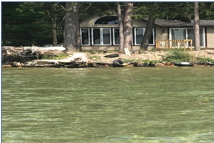
Figure 61. Shoreline erosion around Higgins Lake (August 21-23, 2019).
