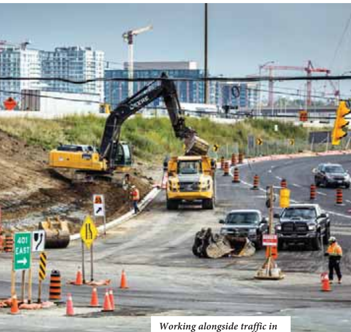
Working alongside traffic in the Highway 401 East project.
