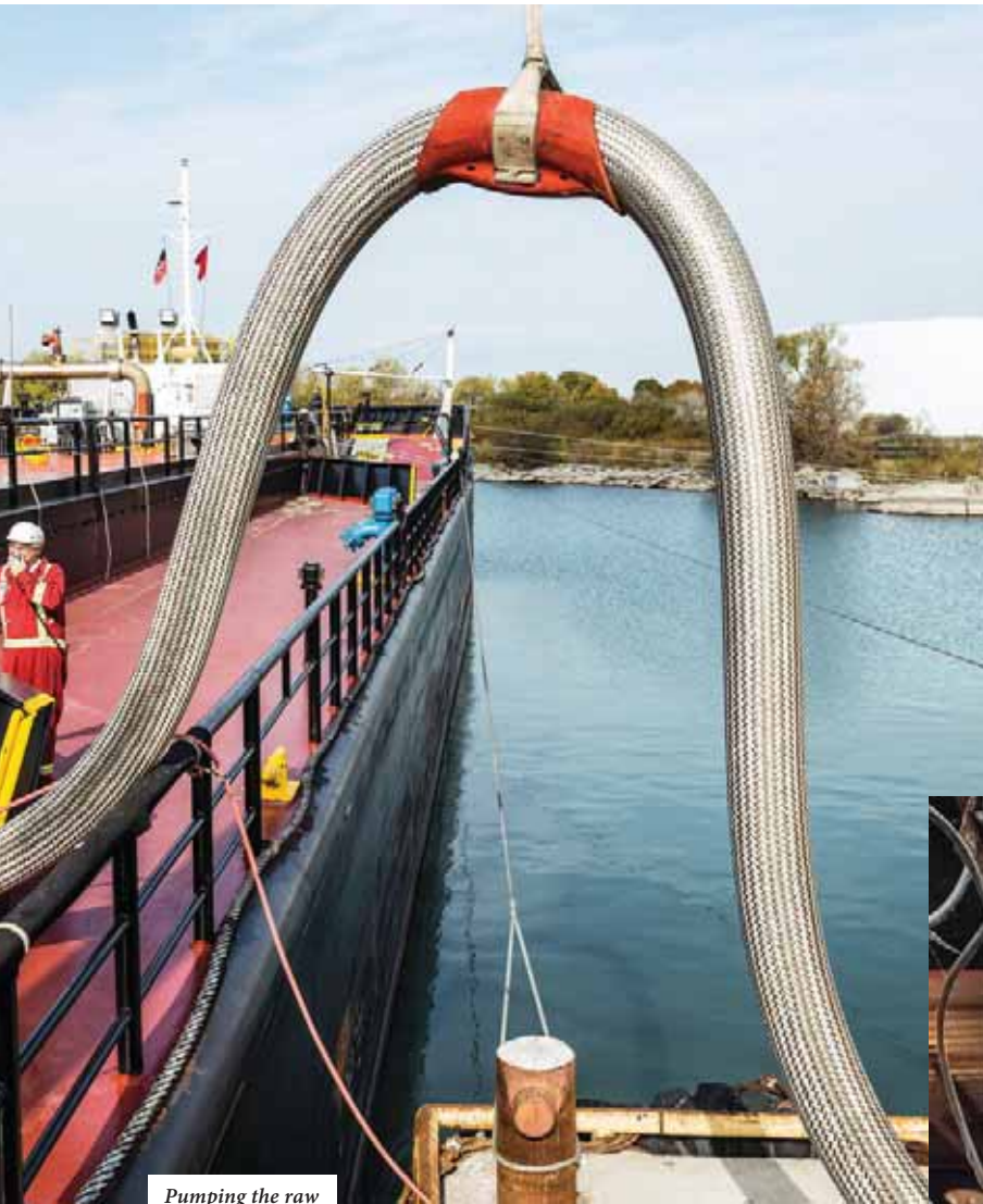
Pumping the raw material to the McAsphalt plant.
