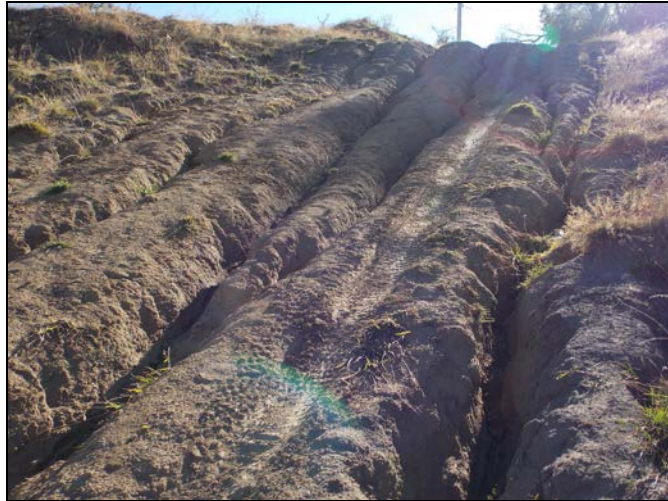
Figure 9: Advanced rill erosion with deep rills.
