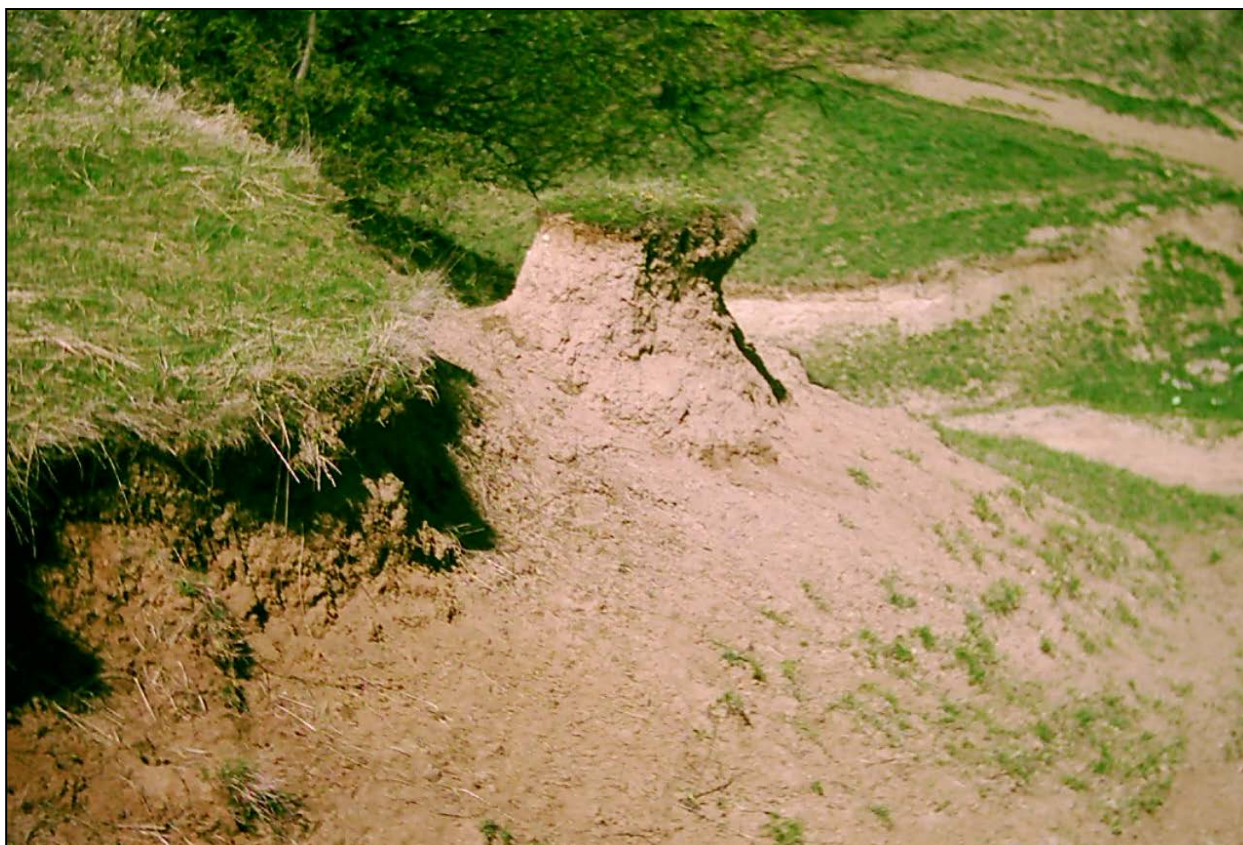
Figure 11: Erosion in surface on the slope due to animal crossings to the pastures.
