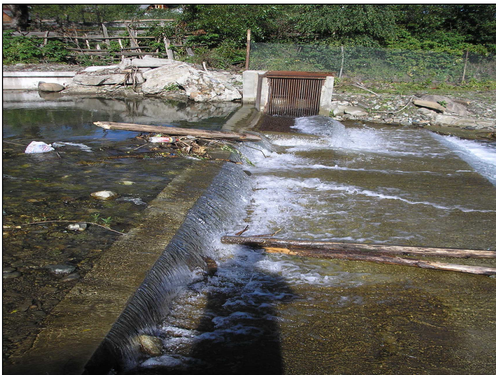
Figure 6: The low level dam from the confluence of the Repede River and the Vișeu River.
