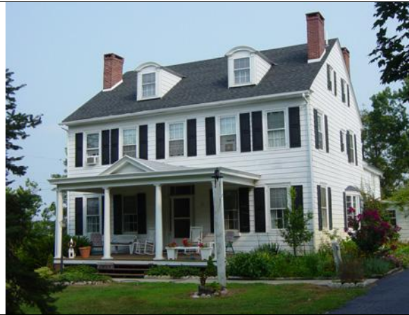
38. 279 Rte 45 Fine federal home which appears to date from the 1 st quarter of the 19 th century. Owned by Andrew Thompson in mid 19 th century. 12 & 13 Porch added, in late 19 th century. Aluminum sided.
