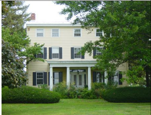
28. 84 Nimrod Road Sarah Bassett Griscom House. Frame Greek Revival house built by Benjamin Bassett for his daughter Sarah and her husband Barclay Griscom about 1854. The original house did not have fireplaces because it was designed to be heated with Franklin stoves. 2 Exterior now covered with aluminum siding.
