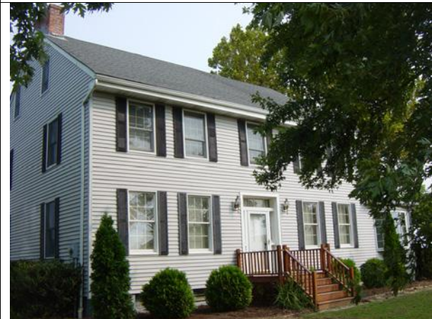
39. 227 Old Kings Highway Frame house probably dating to 1830-1840. Located facing the original route of Old Kings Highway. Now aluminum sided.
