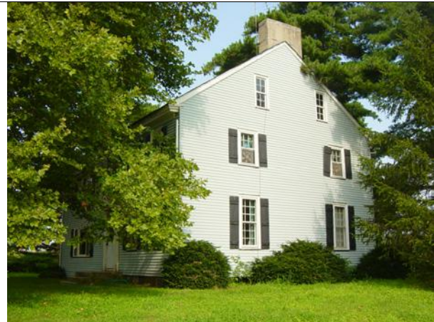
27. Biddle Road Late 18 th or early 19 th century frame house, now covered with aluminum siding. History not known at this time.
