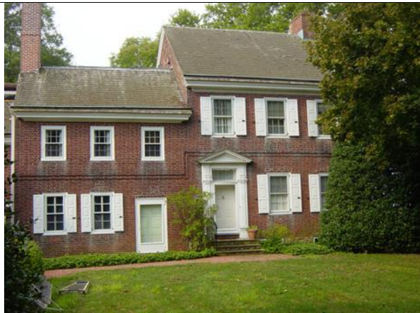
23. 55 Nimrod Road Very fine brick Georgian structure built in 1813 by Jacob Fox. Original exterior including classical front doorway and shutters. Interior retains original chip carved mantels 2 . Modern additions include kitchen to left side, and large room for entertaining to the rear.
