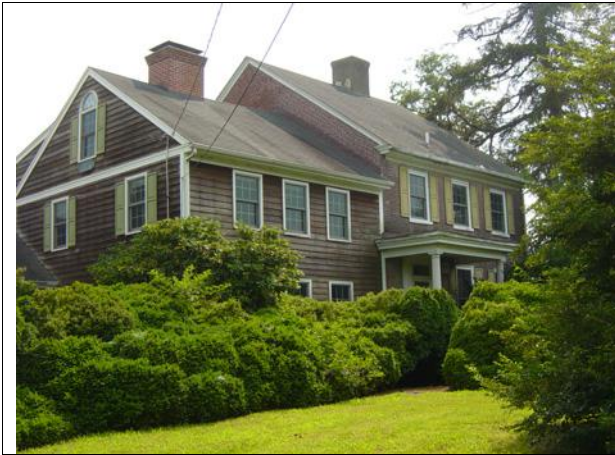
45. 663 Quaker Neck Road Brick section may have been built in the last quarter of the 18 th century. The porch is a later addition. The frame section is dated 1811. The frame section was re-sided in the 1990's. The interior of both sides has been altered.
