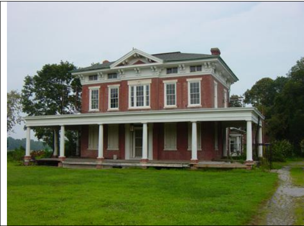
37. 367 Kings Highway Hiresdale: Very fine Italianate brick house. Dated 1865. Named for the Hires family who ran a very successful dairy from this farm.
