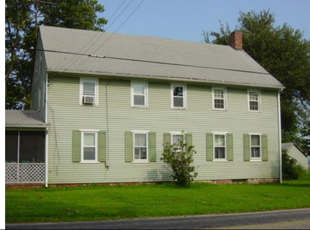
25. 61 Halltown Road Rachel Bassett Allen House. Frame House built around 1855 or 60. Now covered with aluminum siding. Built by Benjamin Bassett for his daughter, Rachel, who married Collins Allen. 2
