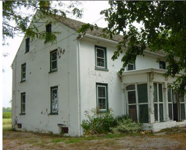
47. 510 Quaker Neck Road Unrestored brick house circa 1775. Brick exterior has been stuccoed. Late porch added. Most of original interior is gone, except for several very nice 18 th century doors on the second floor.
