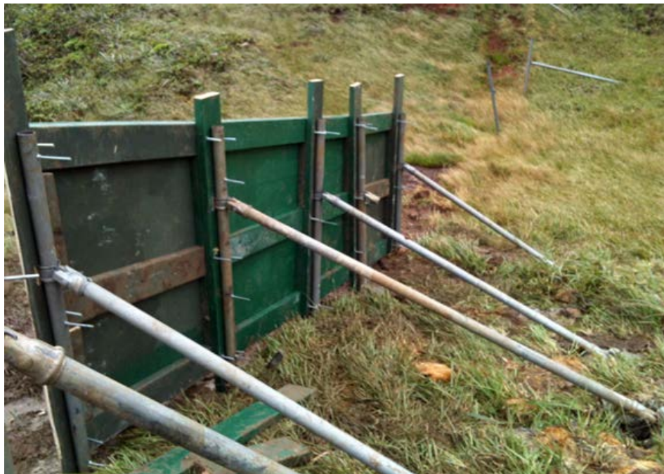
Completed test section of OANRP fence design: 2"x6" framing with 3/4" ply.
