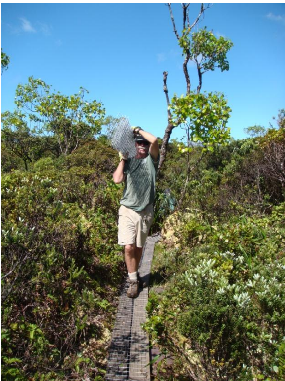
Volunteer hauls wire mesh for the boardwalk improvement project at Kaala.
