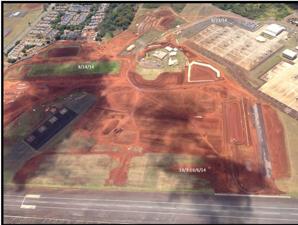
Aerial photo of the WAAF construction site.
