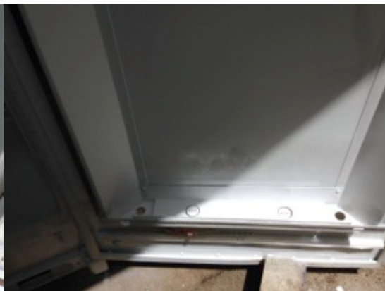
Figure 1. Chamber refurbishing and maintenance. Photo labeled A shows rust penetrating the frame of the chamber, where door hinge failed. Photos B and C depict a typical rusted chamber floor and door with light fixture. We moved the chamber outdoors, treated for rust, scraped with
