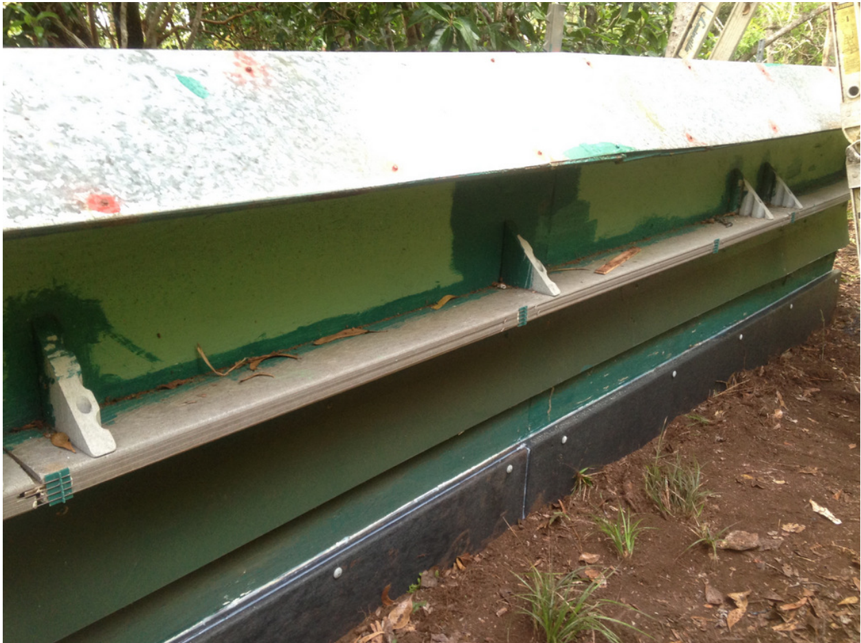
Figure 3. Recent enclosure wall upgrades showing plastic lumber at ground level and wall supports on the inside.
