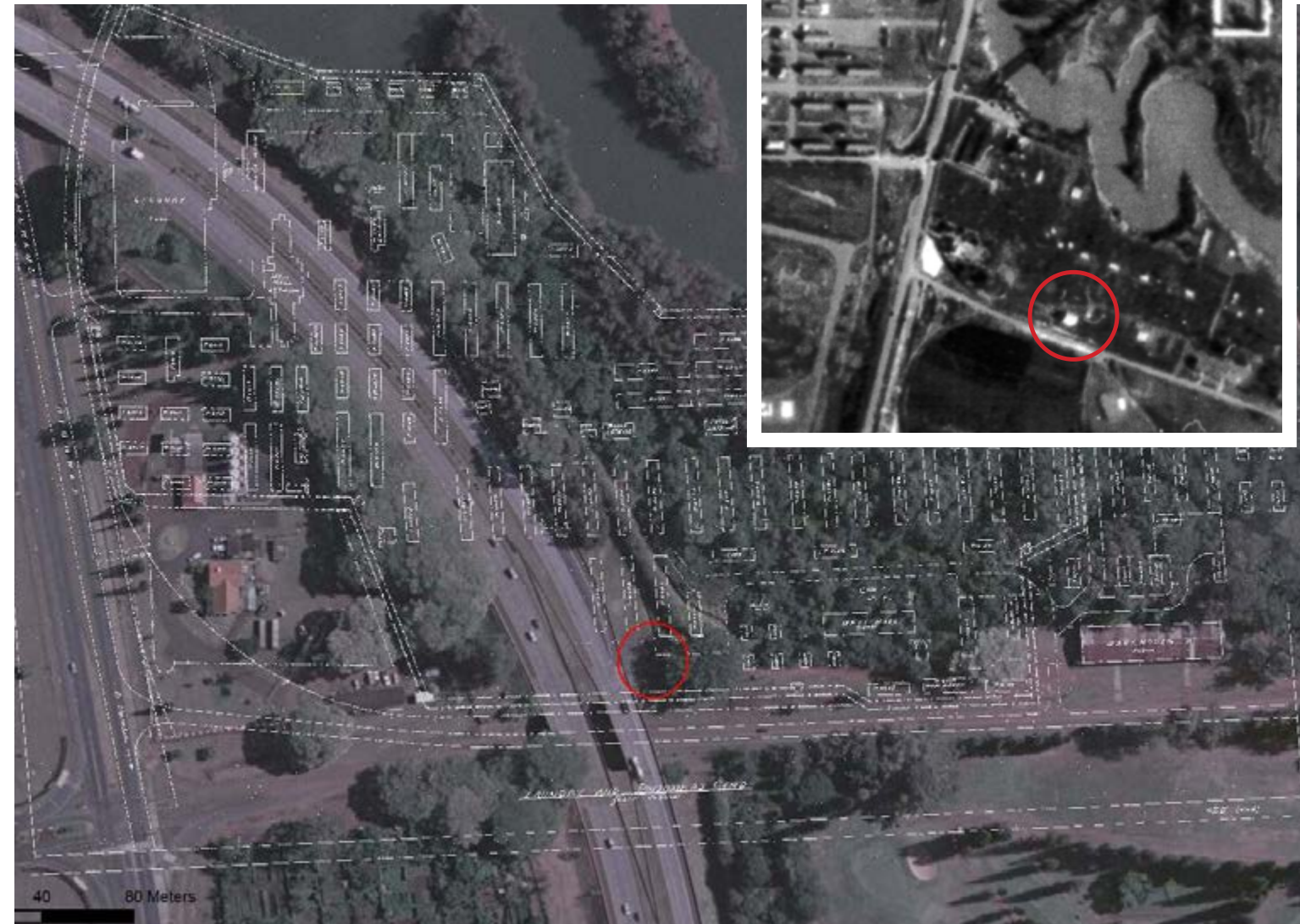
RIGHT A 1948 aerial photo of the POW camp remnants shows Mother Cabrini chapel intact (circled in red). Three years later, it appeared to be a pile of rubble. BELOW Today, the camp stretches across the area below H-2. The location where the chapel would have stood today is circled in red (Google Earth aerial, 2010). IMAGE AND PHOTO BY OACRP
