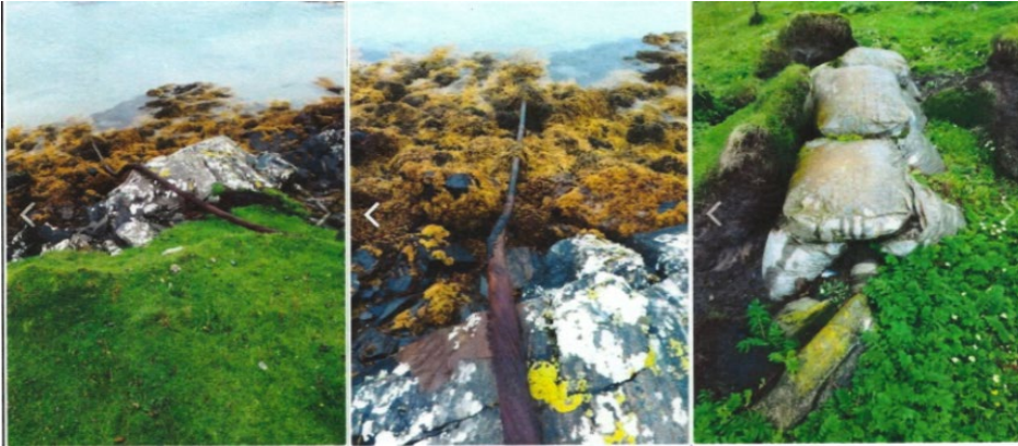
Figure 8- Benbecula shore end, showing exposed cable
