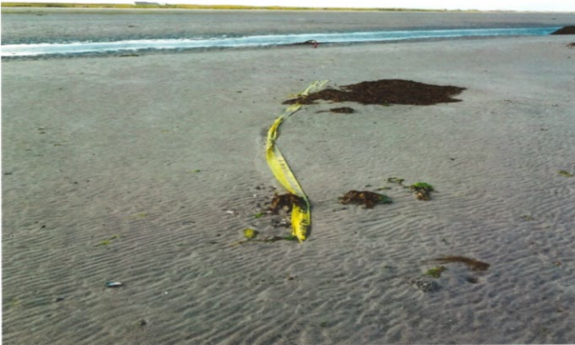
Figure 11- South Uist West shore end, showing exposed cable tape
