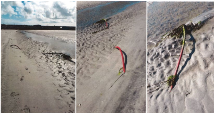
Figure 10- Benbecula shore end, showing exposed cable
