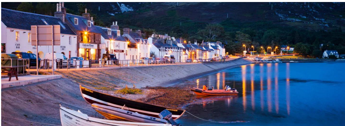
Figure 4.1: Shore Street Revetment
