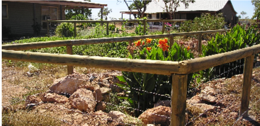
Figure 12. Wastewater Gardens at Joy Springs (Eight Mile) Community, Fitzroy Crossing, West Australia include gravity-flow and inverted leachdrains for wet season operation. (a) The Wastewater Gardens are long and narrow, 1m x 12m, to fit into old leachdrains which were dynamited through hard underlying rock. (b) The inverted leachdrains were planted with a variety of native and decorative/useful plants and is watered by treated effluent during wet periods of the year and has a reticulated drip irrigation system as well. (c) both Wastewater Garden and inverted leachdrains are fenced with low wooden post and rail and mesh to exclude children, dogs and grazing animals.
