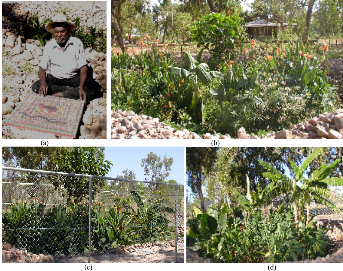
Figure 10. Three Wastewater Gardens at Emu Creek community, Kununurra, West Australia, with areas of 48 m 2 , 30m 2 and 24m 2 treat the wastewater of the entire community. They have solved long-term problems with exposed sewage and failure of house plumbing due to high groundwater during the wet season. Control box covers were painted by community residents to increase stakeholder participation (a) Ned Johns with painting of snake and emu (b) combined WWG that serves two lowest houses (c) and (d) gardens behind cyclone fences erected one year after installation.
