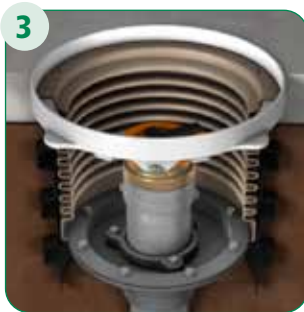
3 Replace Bellows, Reinstall Upper and Lower Rings
