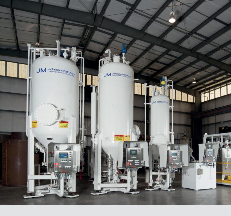
When refilling, carrier air is usually vented to atmosphere. To prevent any fines escaping, the **INTERCAT** loader is fitted with a sintered metal filter (SMF). This is a stainless steel mesh self-cleaning system which prevents any powder escaping the addition system during refill. There is a back pulse system that cleans the filter while in operation and blows back the fines into the vessel.
