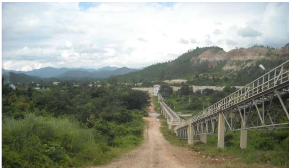
Figure-9: Conveyor line
