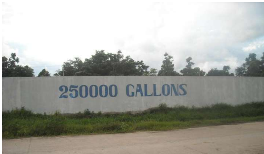
Figure-16: Water storage tank
