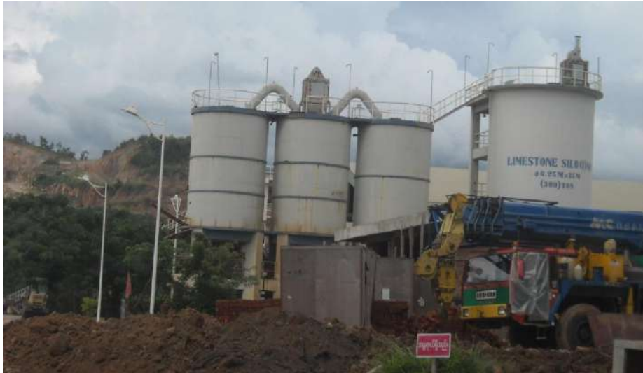
Figure-10: Limestone silo
