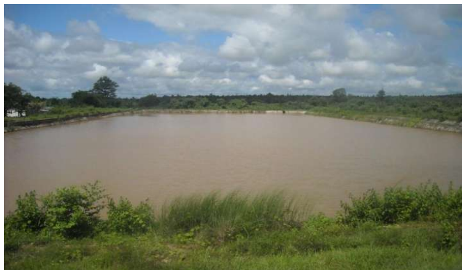
Figure-17: 3 million gallons weir
