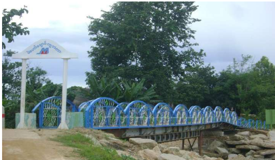
Figure-41: Mei-hor Bridge
