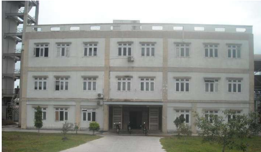
Figure-7: CCR building
