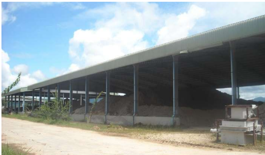
Figure-15: Shed for mined out materials
