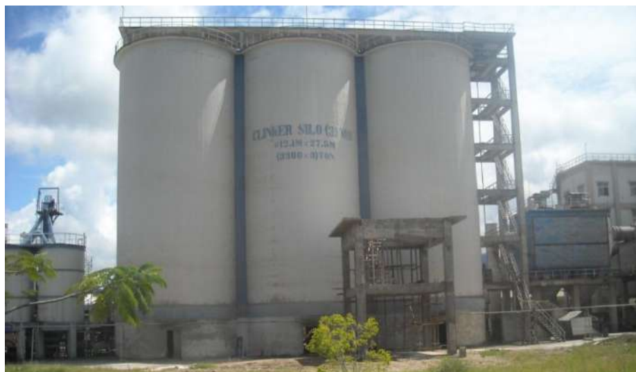
Figure-12: Clinker silo
