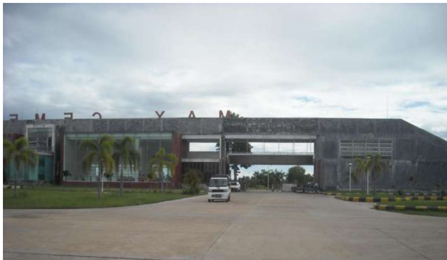
Figure-5: Main building (office is on the left side)
