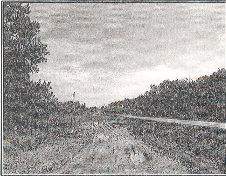
VIEW FROM SUBJECT EAST ALONG SPRING CYPRESS
