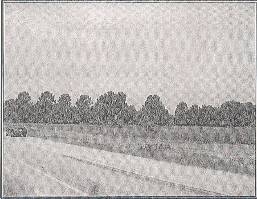
VIEW OF EASTERN PORTION OF SUBJECT PROPERTY
