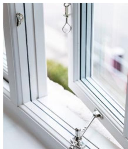
In Fabriken1891 (Hermes 10) in Helsingborg, parts of the property were fitted with new energy-efficient windows that are similar in appearance to the original windows. In Henry Dunker's office, windows and sashes were specially ordered and stained brown on the inside to harmonise them with the panels. Much of the other original interior fittings have been preserved, such as the herringbone parquet, the dark wainscot and a built-in vault.
