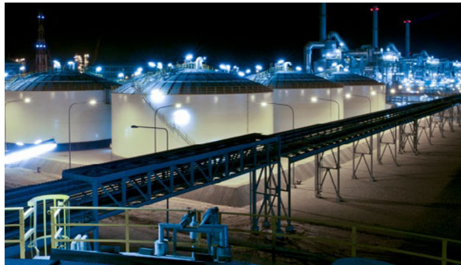
The world's largest sulfuric acid plant complex was built for Ma'aden in Saudi Arabia using Outotec technology. Ma'aden will also use Outotec-Hatch technology in its aluminum plant project.
