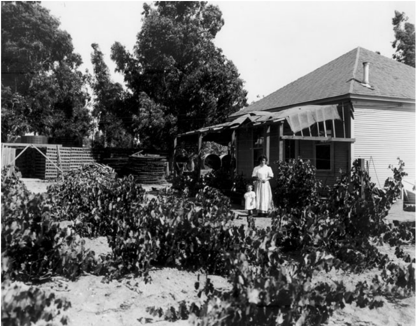
Guasti, ca. 1910. Italian woman and girl in front of one of the houses the Italian Vineyard Company offered to workers with family. Before Prohibition, company housing was reserved to Italians. Japanese and Mexican temporary workers camped outside town, across the Southern Pacific Railroad. Courtesy Cal Poly Pomona University Library Special Collections.
