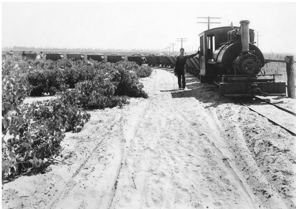
Italian Vineyard Company, Guasti, ca. 1910. The narrow-gauge train used to transport grapes from the vineyards to the winery. The movable railroad was necessary because of the extension of the vineyards and the sandy soil, which made the use of draught animals difficult. Courtesy Cal Poly Pomona University Library Special Collections.
