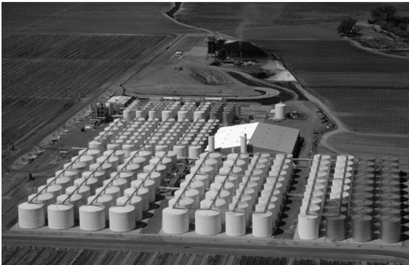
A large plant for wine storage and fermentation of the E. & J. Gallo Winery at Livingston, California, ca. 1972. Courtesy Corbis.
