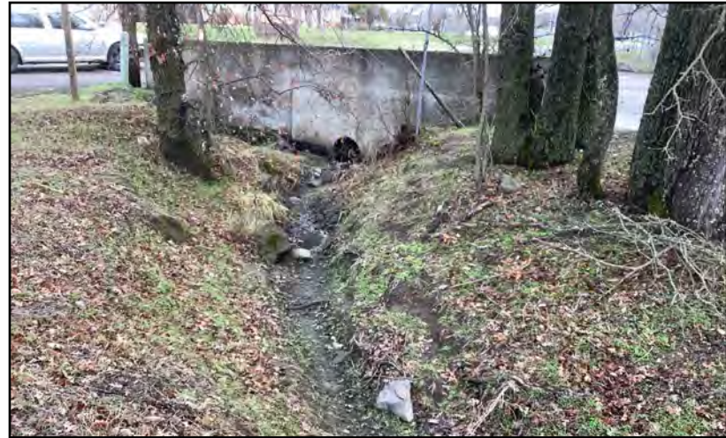
Photo 2. Culverted inlet for the onsite drainage located in the northeast corner of the Study Area. Photo taken January 29, 2021, facing west.
