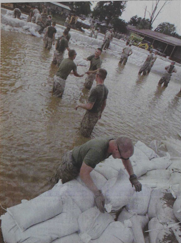
Marines and sailors of 26th Marine Expeditionary Unit stack sand bags to reinforce the levees. Cpl. Jason D. Mills
