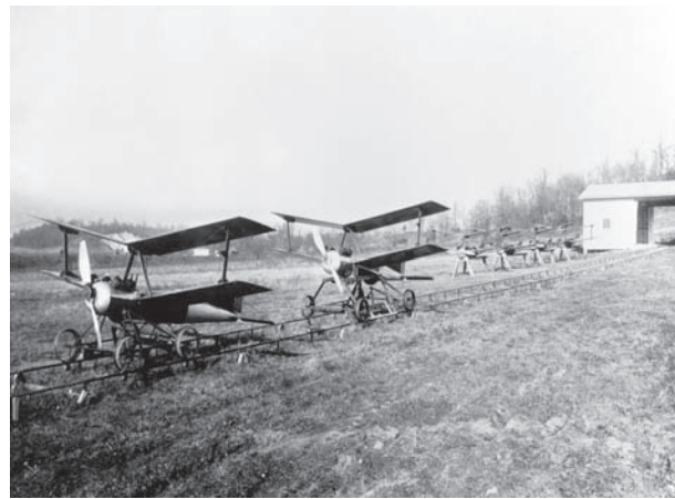
Figure 3. Kettering "Bug" The first mass produced guided weapon.
