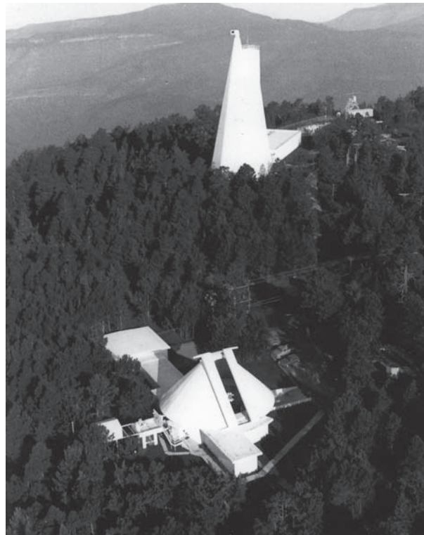
The Sacramento Peak Observatory includes the Solar Vacuum Telescope (top), which features a 220-foot vertical shaft and a connecting laboratory building. The site also includes a 16" coronagraph and a 12" coelosts telescope for solar observation.
