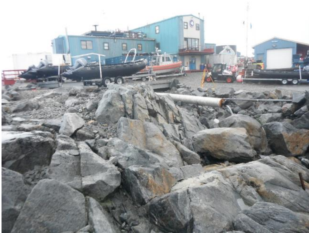
Description: Existing sanitary sewer outfall
