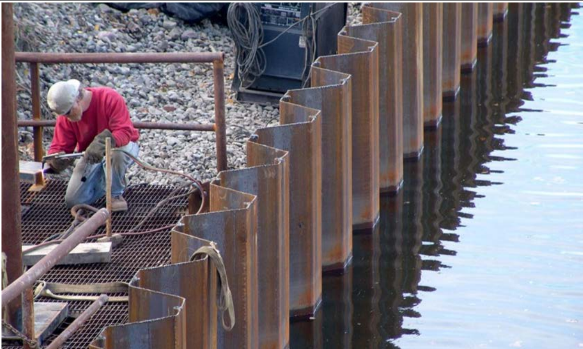
Description: Waterfront installation of sheetpiles
