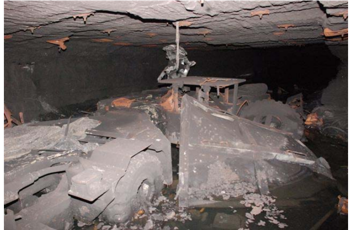
A scoop located on the Headgate 22 section after the April 5 explosion
