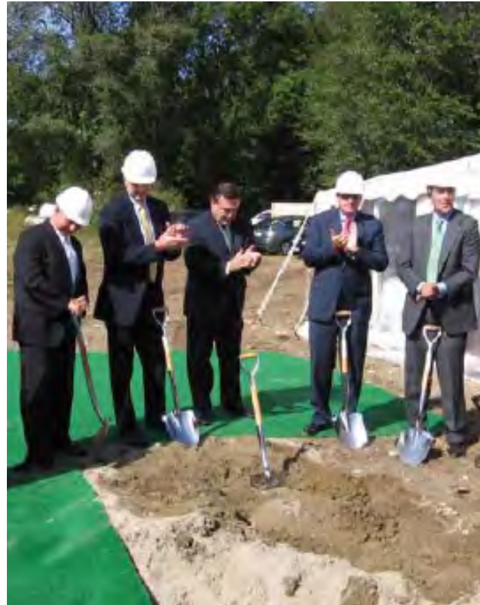
The first incursion of OHL into the U.S. market occurred through Inima, the Group's head company for environmental activities. It was the first Spanish company to contract a desalination plant in the United States, in Brockton, Massachusetts. The cornerstone laying ceremony was attended by (in the photo, from left to right): Jack Yunits, Mayor of Brockton; Jeff Hanson, partner of Bluestone; Marc Pacheco, Senator for the State of Massachusetts; Pedro Mejía, Secretary of State for Trade and Tourism of Spain, and Mariano Aisa, Deputy Chairman of the OHL Group.
