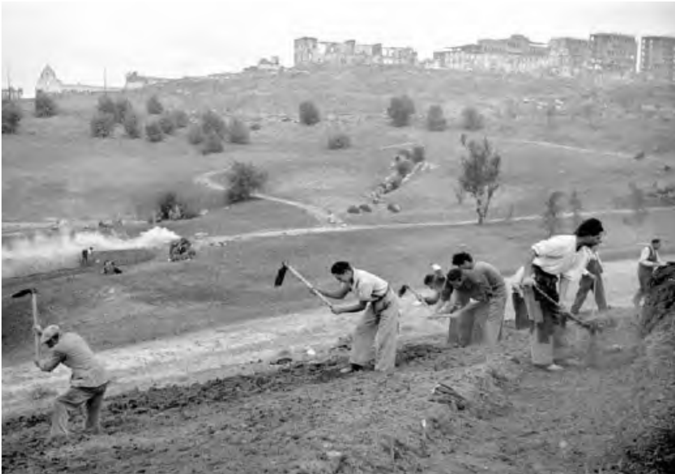
Reconstruction work in the post-war era. In the photograph, reforestation in the gardens of the West Park.
