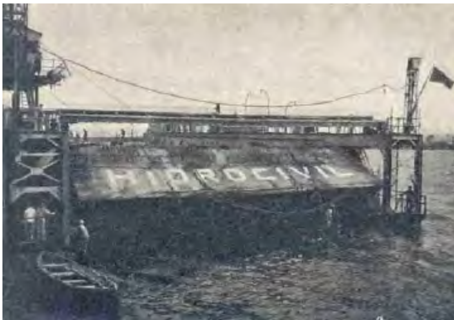
At the end of the twenties, Obrascón undertook a number of large-scale projects, such as the Nuestra Señora del Rosario dry dock at the Port of Cadiz. The launch, in 1929, of the first of the 13 caissons of the dock was a technological milestone. It was the largest built in the world up to that time, weighing 3,200 tons.
