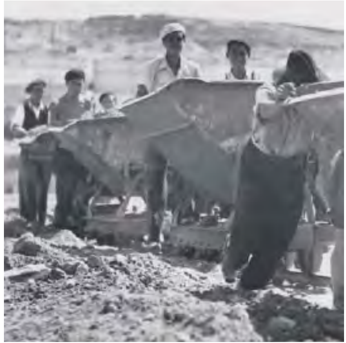
Dumpers pushed by workers for the transport of material were a routine resource in construction work during the thirties.
