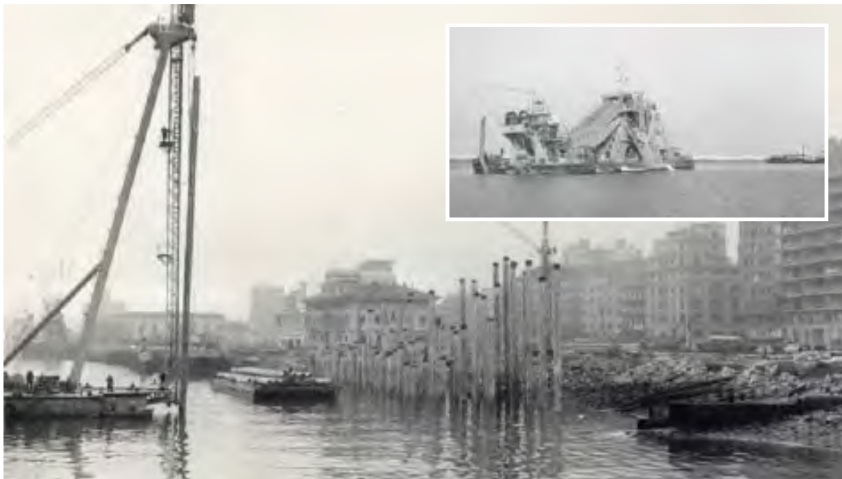
In the fifties, Obrascón remained focused on its traditional civil engineering market, with the predominance of port construction. In the photographs, one of the crane pontoons used by the company during that decade for moving large volumes of material at its work sites and Cubipods at the Rota Naval Base in 1959. Below, construction at the Port of Santander in 1967 and dredging in the Port of Cadiz in 1962.
