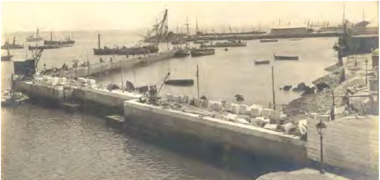
1913 was prodigal in winning contracts, such as the awards of the construction of dock 1 of the Reina Victoria wharf at the Port of Cadiz, whose construction and completion are reflected in the photos. It was formally dedicated in 1920.
