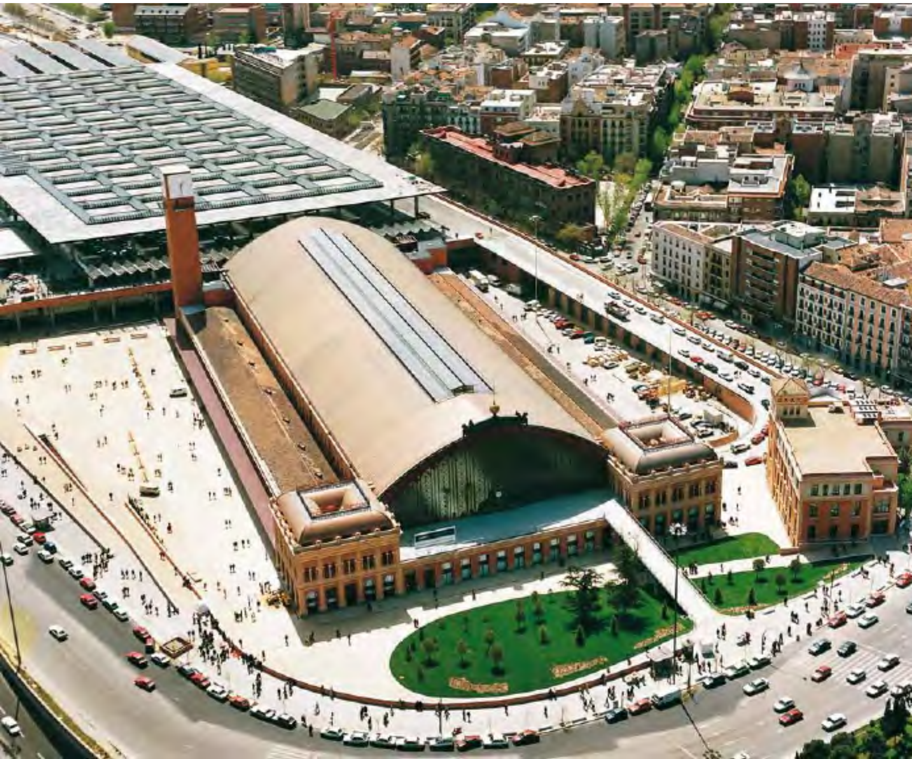
Atocha railway station: the reconstruction works for accommodating the head shunt of the Madrid-Seville AVE railway line were completed in 1992.
