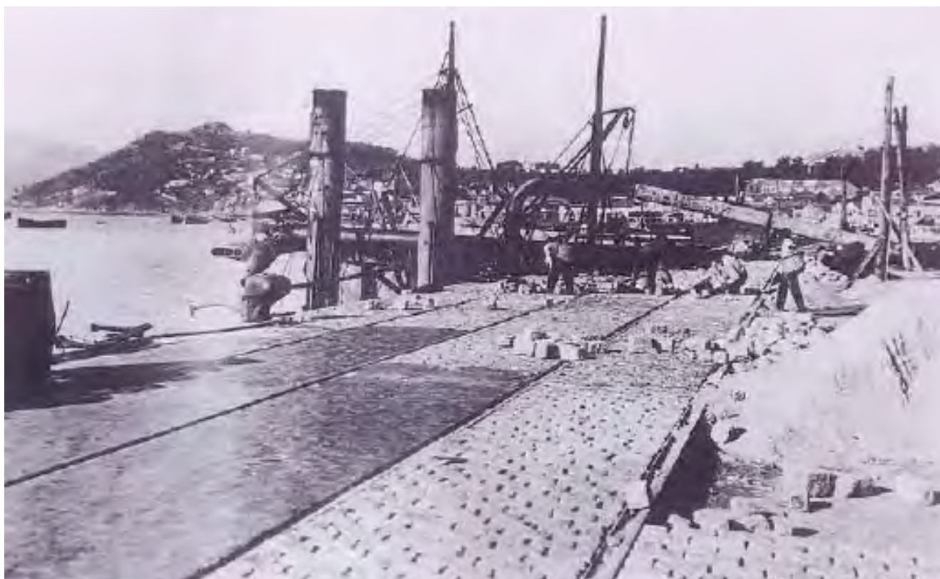
These two photographs show the construction of the Ribena de Areal wharf in Vigo. Above, a side view and, below, the tracks and pavement: both were works performed by Obrascón in the thirties.
