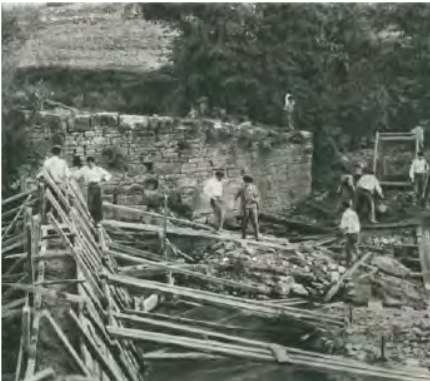
Brigades of workers in the construction of the Urdaniz Dam in Navarra, during the thirties.
