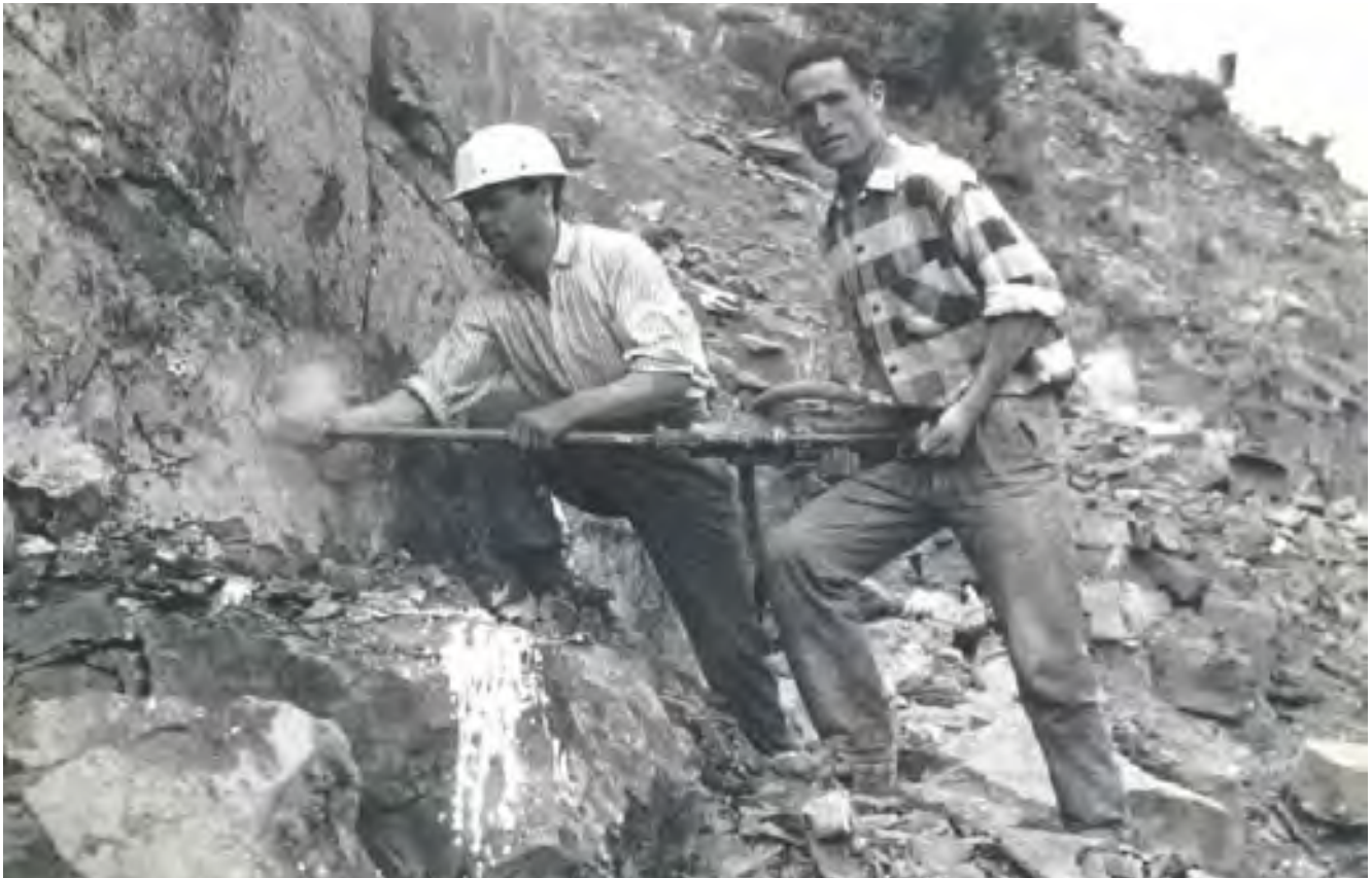
Workers in an Obrascón quarry in the forties.
