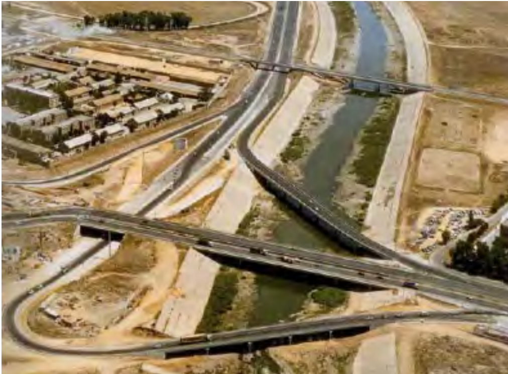
64% of the new contracting secured by Obrascón in 1990 referred to civil works, as the most outstanding business line in the entire backlog. To the left, East Bypass II in Seville.
