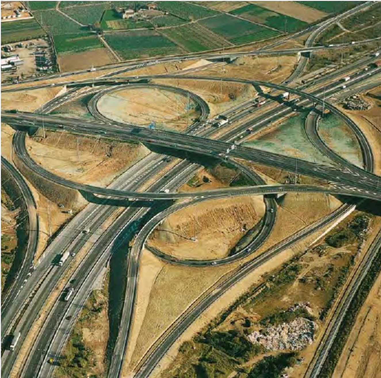
South leg of Barcelona's Coastal Beltway.
