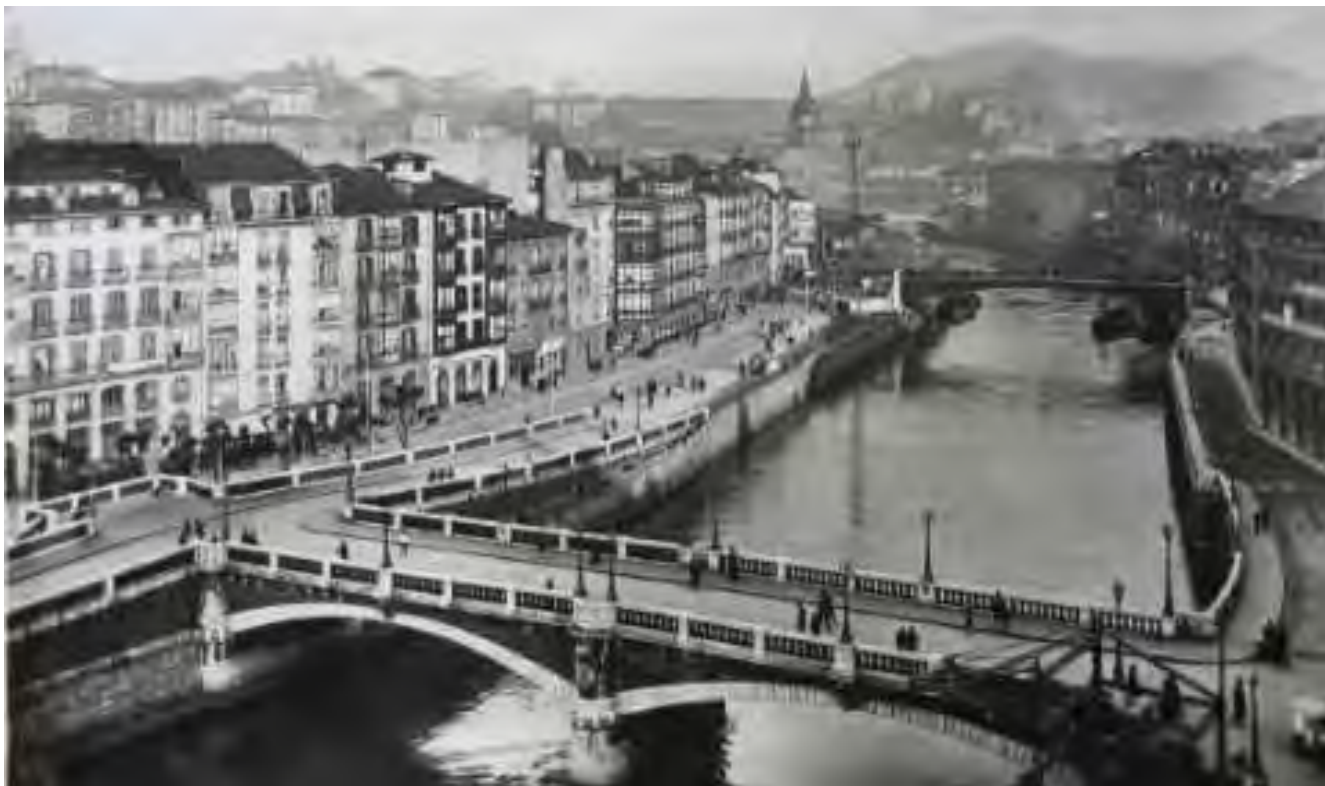
In 1937, Obrascón's Board of Directors decided to take part in the call for tenders by the Town Council of Bilbao for the construction of the General Sanjurjo Bridge, to replace the La Merced Bridge destroyed during the war.
