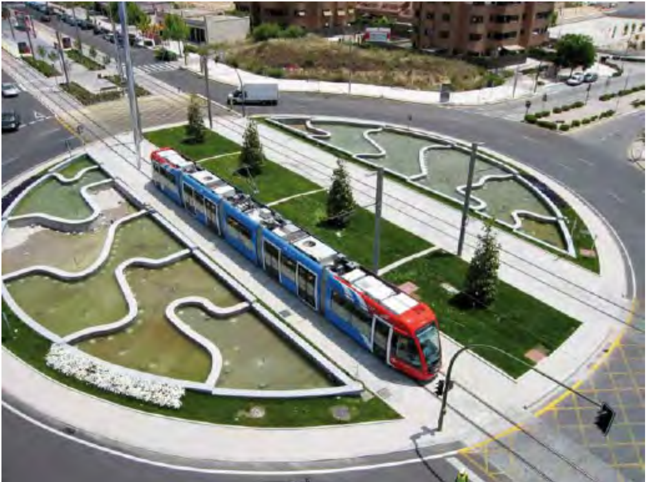
Metro Ligero Oeste is an OHL Concesiones subsidiary that combines business with a new experience in non-polluting intermodal transportation.
