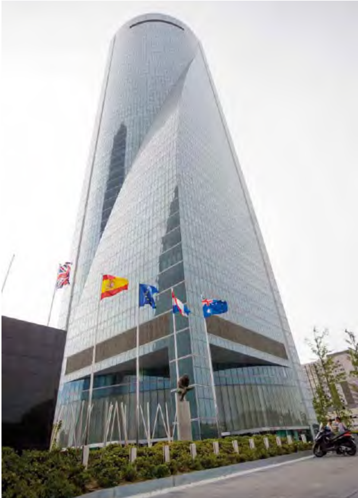
OHL's central headquarters is a manifestation of the future projection of a construction and services group. It integrates the most advanced construction technologies, is home to a highly international community of tenants, including several foreign embassies, and is an icon of modernity in Spain's capital.
