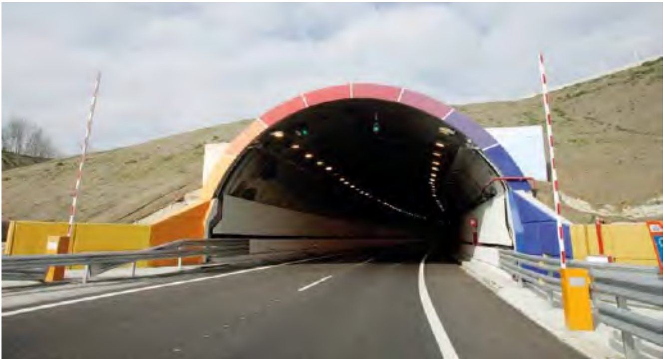
The Eje-Aeropuerto or M-12 airport access toll road in Madrid included supplementary civil works for improving mobility in the areas on the outskirts of the city, mainly with respect to the accesses to the various terminals of the airport. The tunnels built in relation to these works were executed by using the so-called “Madrid method” and have received awards as the best and safest tunnels in Europe.
