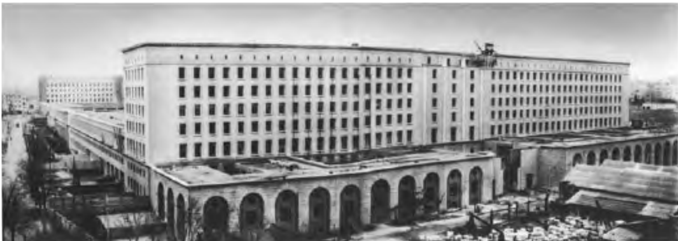
Construction of the Nuevos Ministerios government office buildings by Huarte. Progress of the work in the forties.
