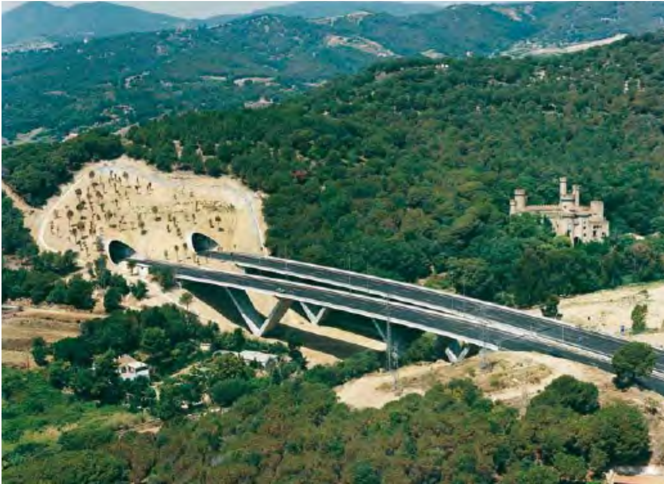
A-19 freeway in Barcelona, one of the most outstanding civil engineering projects performed by Obrascón in the seventies.
