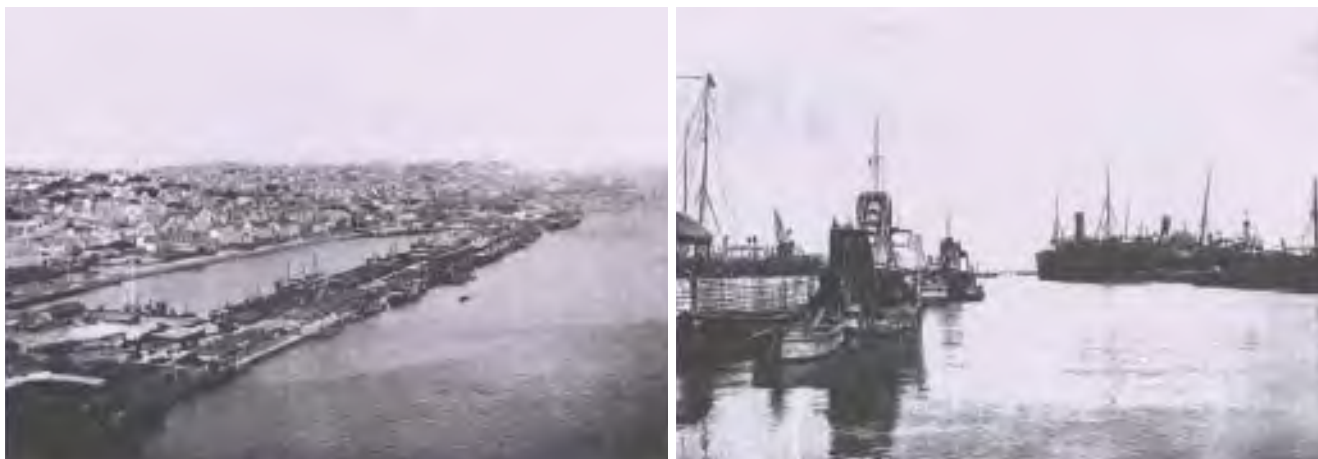
The "Alcántara Dock", Port of Lisbon, and the "Port of Santos West Wharf", also in the Portuguese capital, were the first contracts obtained by Obrascón. Awarded in March 1912 and completed in 1918 and 1915, respectively.
