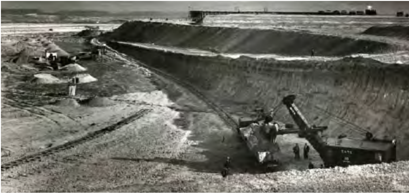
Earth works for Madrid's Barajas Airport in 1945, performed by Sato.
