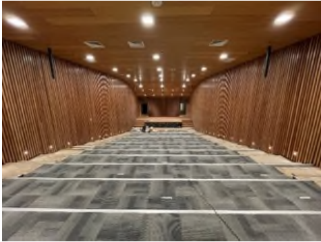
Assembly hall of the Central Crime Lab (PDI), Chile.
