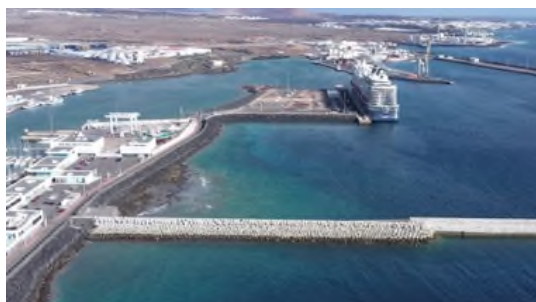
Cubipods. Naos southern outer sea wall cruise ship dock. Port of Las Palmas, Canary Islands. Spain.
