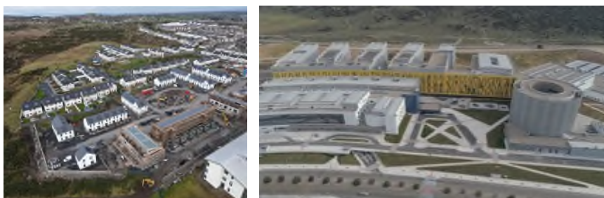
From left to right, PPP housing units in Ireland and the Toledo University Hospital (CHUT) in Spain.
