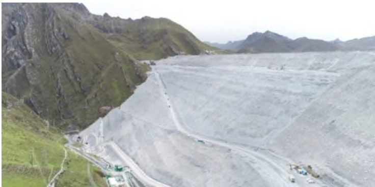
Antamina tailings dam, Peru.
