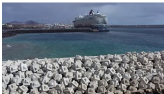
Cubipods. Naos southern outer sea wall cruise ship dock. Port of Las Palmas, Canary Islands. Spain.
