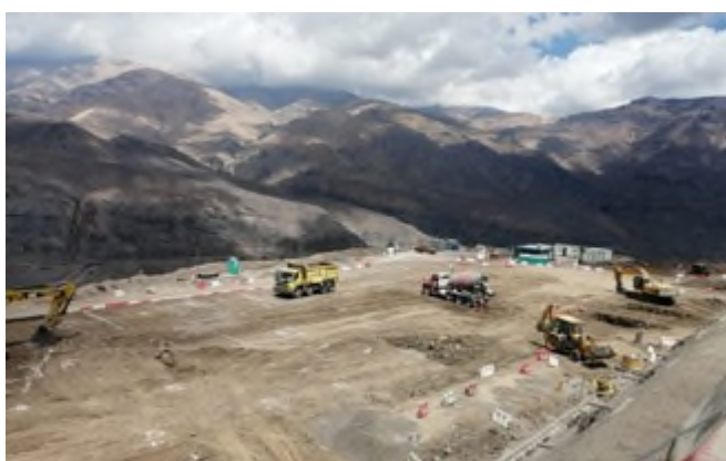
Earthworks at the Teniente mine, Chile.
