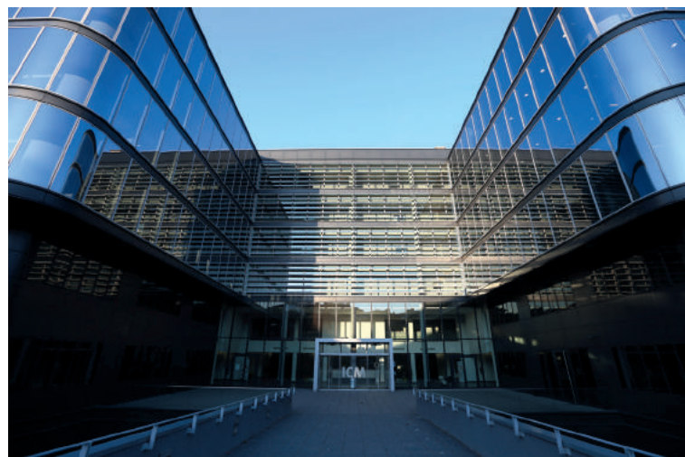
The building's characteristic H shape promotes a maximum of exchange among the research teams working on site
