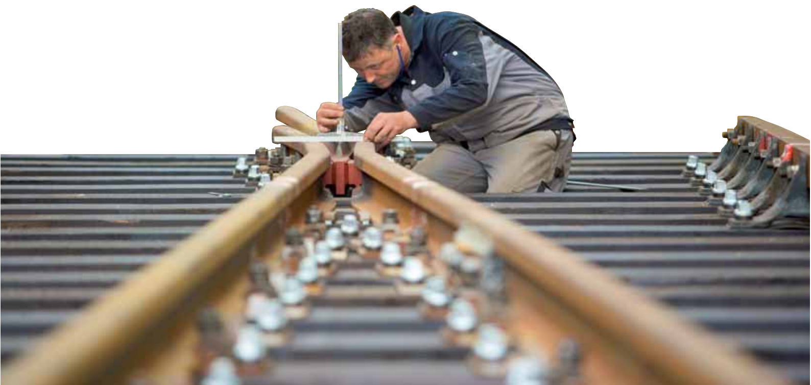
Precisely! A Vossloh switch being put into place.
