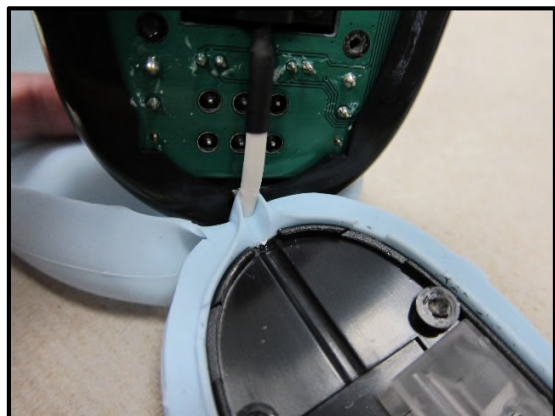
Figure 16: Cable penetration is dry
