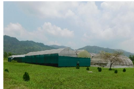
Outer view of Polyhouses
