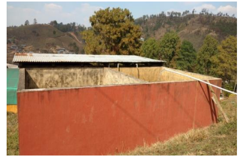
RCC Water Reservoir
