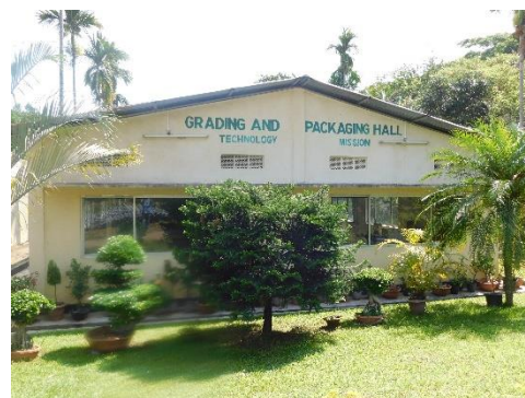
Grading & Packaging Hall
