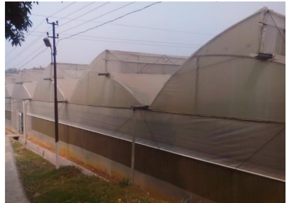
Outer view of Polyhouses
