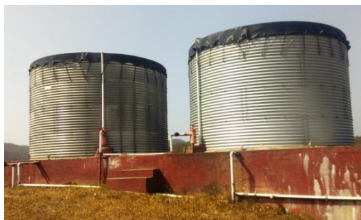
Genap Water Reservoir
