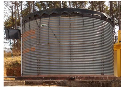
Genap Water Reservoir
