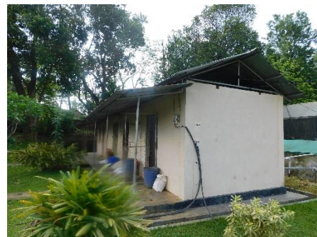
Security & Fertigation House
