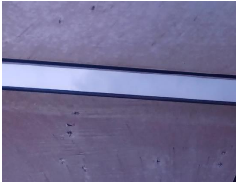
Holes in Polyhouse roofs repaired with cellotape
