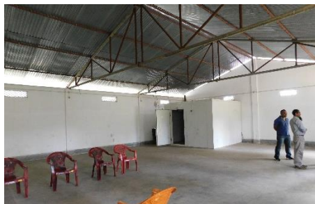
Cold Chamber (left in the picture above) and Grading Hall
