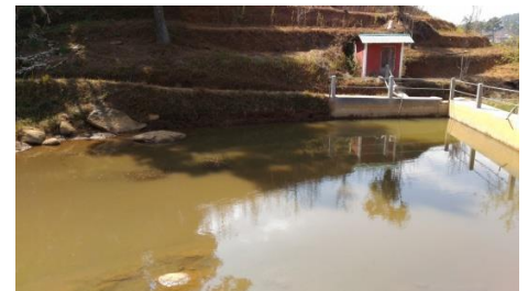
Water Harvesting Pond & Pump House
