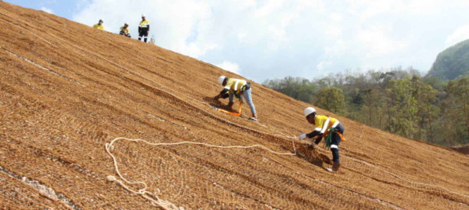
Memasang jaring sabut kelapa ( coconet ) sebagai fondasi penanaman pohon di lereng bukit di Wetar. (FOTO: BKP-BTR) Installing coconut cair (coconet) as a foundation for planting trees on the hillside in Wetar.
