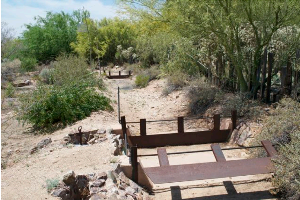
Fig. 44 Channel with gates to control the flow of water
