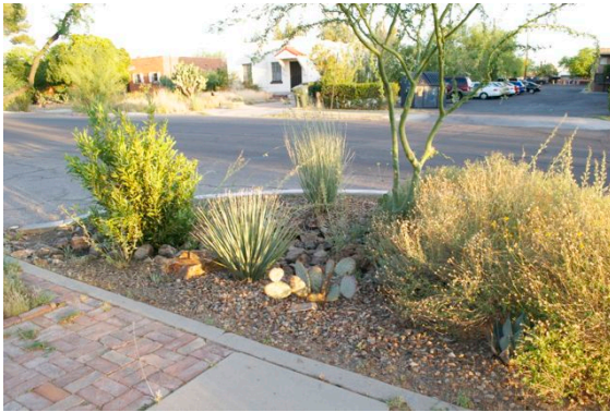
Fig. 48 Curb cuts and basins at road intersection
