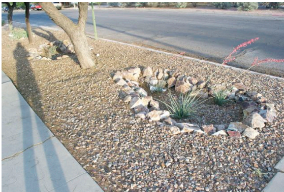
Fig. 50 Berm and gravel filled trench
