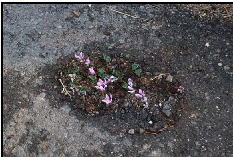
Figure 106 A tenacious plant with difficult digging conditions!
