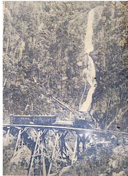
Original trestle bridge across the creek, at the base of the waterfall. Photograph of interpretation sign
