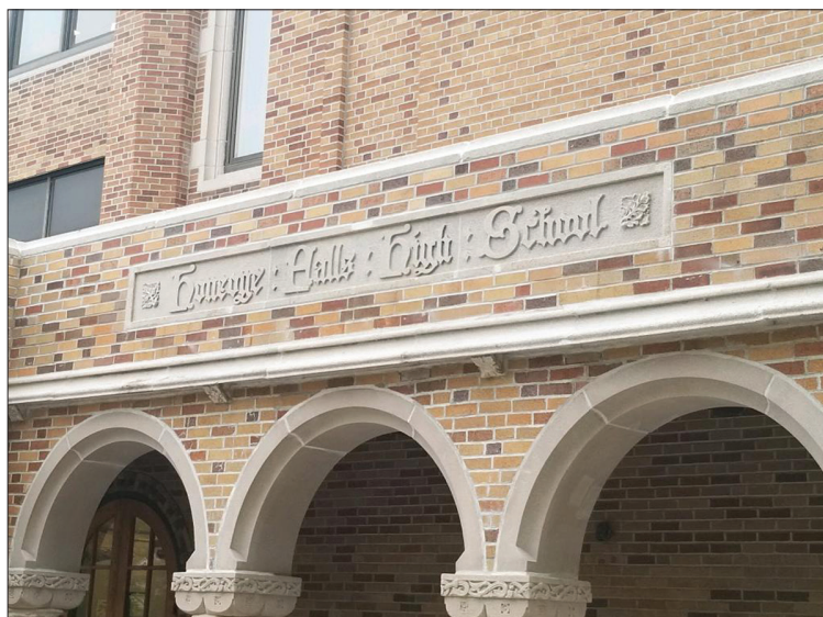
The restored facade at HF-L high school. Submitted photo
