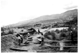
18 Feb. 1939. North Argentina, prov Jujuy, between Tilcara and Humahuaca; low bridge washed away by flash floods, and workmen repairing damaged railway line.
