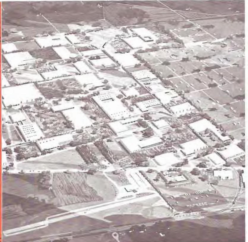
Artist's rendering of the 610-acre industrial park at suburban Schaumburg, Ill., indicating how the area will appear when developed. The Milwaukee Road, which will serve the park exclusively, sold it to Centex Corporation in 1969.
